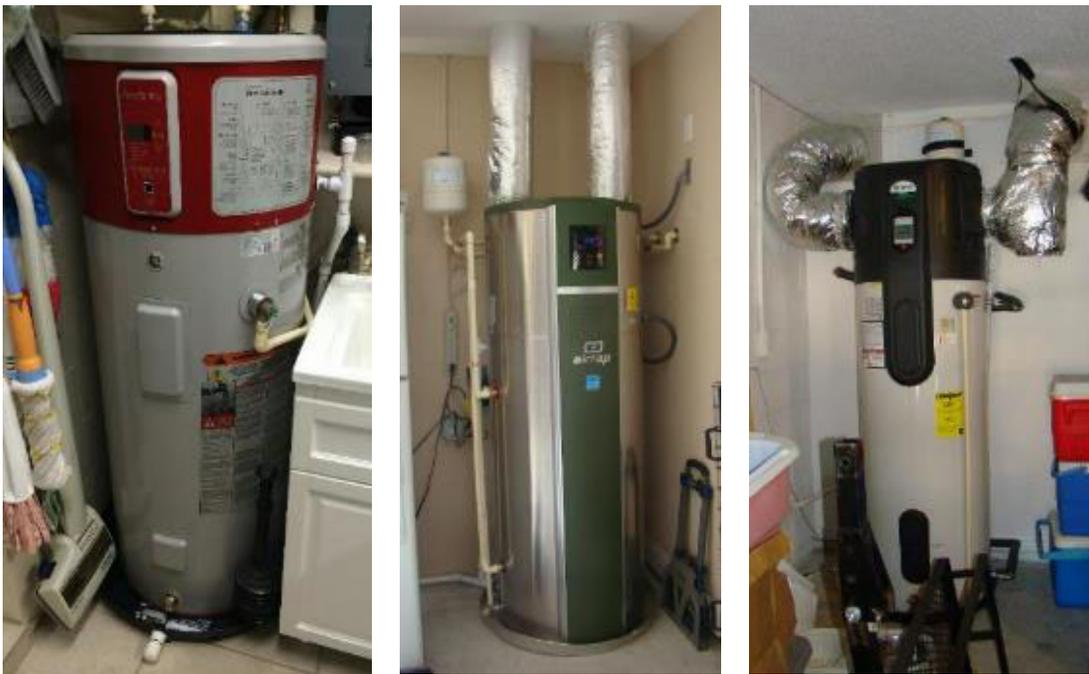
Figure 4. HPWH configurations: Left, interior GE unit in utility room, Site 13; center, ducted Airgenerate unit at Site 5; right, ducted A.O. Smith unit at Site 26.
