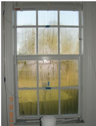
Figure 6. Unvented tight house north-facing window condensation January 23, 2013.
