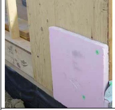
Figure 4. XPS foam at corner
