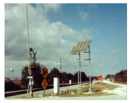
Figure 3-17. PV-powered railway signals (FEC).
