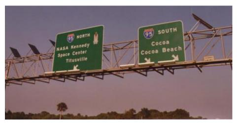
Figure 3-6. PV-powered guide sign lighting, Brevard County, FL (FDOT).
