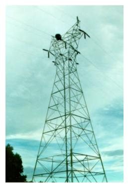
Figure 3-15. Transmission tower beacon powered by PV in the Florida Keys.
