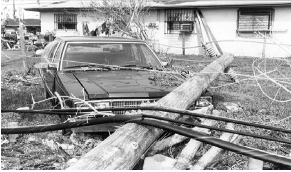
Fig. 1: Utility pole destroyed by Hurricane Andrew
