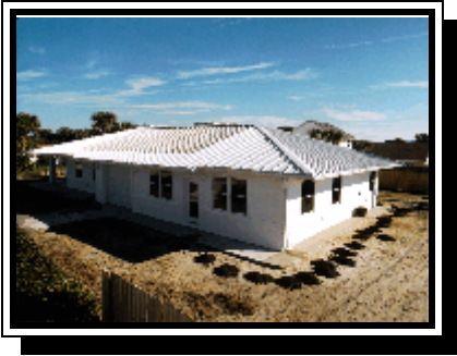
Figure 12. A residential PV system in New Smyrna Beach
