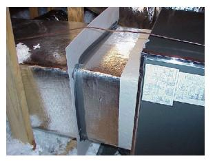
It was not appropriate to cut through the supply plenum in a number of homes, either because there was insufficient space around the plenum, or because the supply plenum was a flex duct. In those cases, the entire duct system was tested. When the entire duct system had to be tested, test pressures were measured in parts of the supply and return ducts as well as in the air handler.
