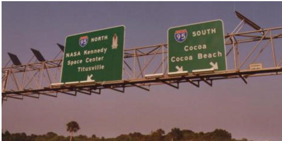
*Figure 3-6. PV-powered guide sign lighting, Brevard County, FL (FDOT).*
