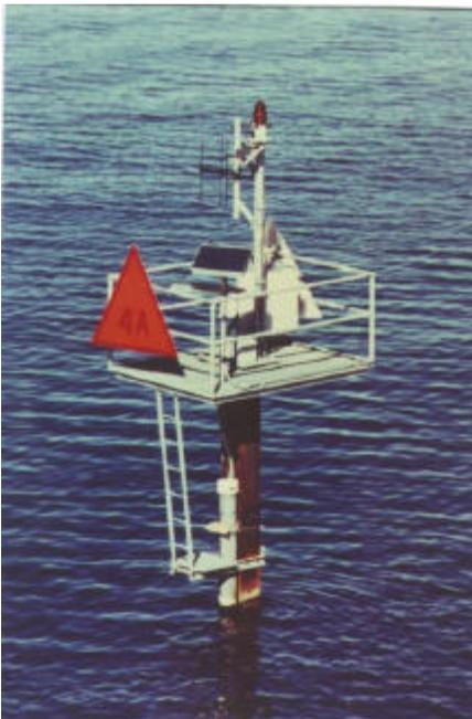
*Figure 3-12. PV-powered flasher on navigational aid, Kissimmee River, FL (SFWMD).*
