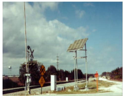
**Figure 3-17. PV-powered railway signals (FEC).**
