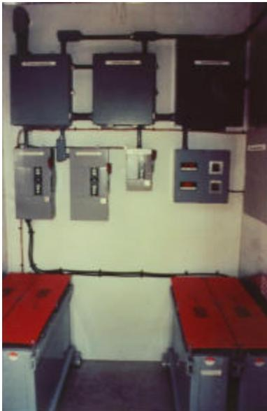
*Figure 3-5. Guide sign lighting battery and control room.*
