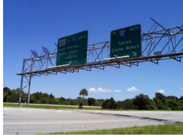
Figure 3-2. PV-powered highway guide sign lighting system.
