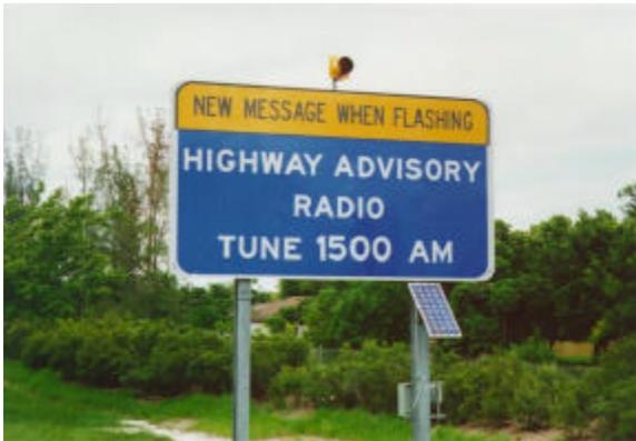
**Figure 3-14.** PV-powered flashing light on Interstate 75, Broward County, Florida (FDOT).
