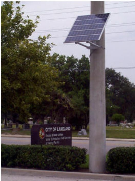
**Figure 3-10. Internally-illuminated PV-powered sign (Lakeland Electric and Water).**
