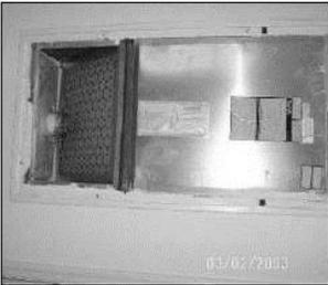
1 AIR HANDLER SEALED TO DRYWALL. SEAL MADE WITH MASTIC AND AIR HANDLER WITH FABRIC.
