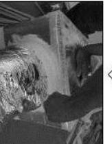
14 SEAL OUTER LINER TO DUCTBOARD WITH MASTIC TO PREVENT CONDENSATION
