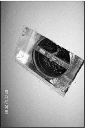
2 CAULK ALL FIRE DAMPERS WITH SHEET ROCK BOARD, PROVIDE 1/8\"
