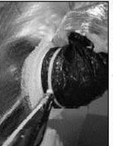
12 SECURE FLEXDUCT INNER LINER TO TENSIONER TOOL
