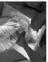
13 ADD ADDITIONAL STRAP TO TOP WITH MINIMUM INSULATION
