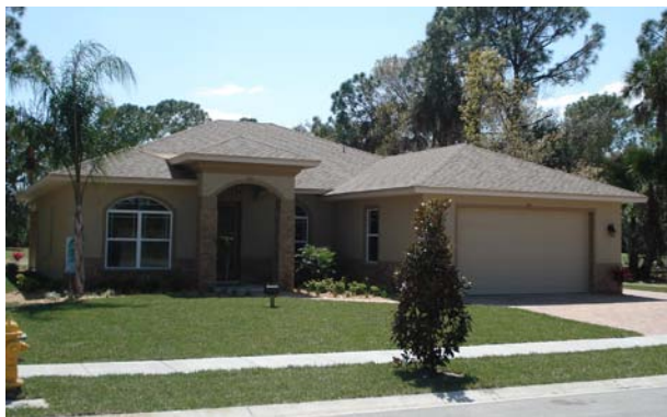
Figure 1: Builder’s Challenge home (2127 Sq. Ft.) construction with conventional hip roof and shingles in Rockledge, FL.
