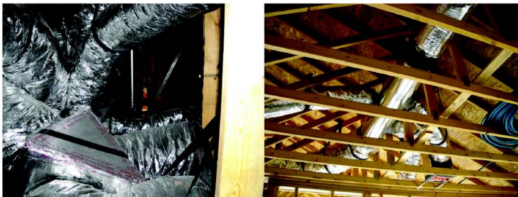
Figure 3 Images of hub and branch ducts (left) and tapered ducts (right).
