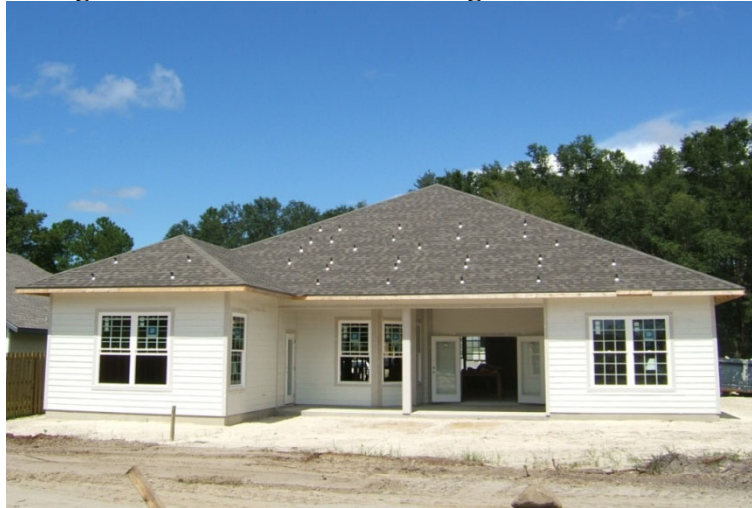
Figure 2. Home at Dried in Stage of Construction
