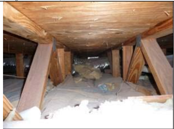
Figure 10 Photo of image above. The floor space is between conditioned space above and below. (Withers)
