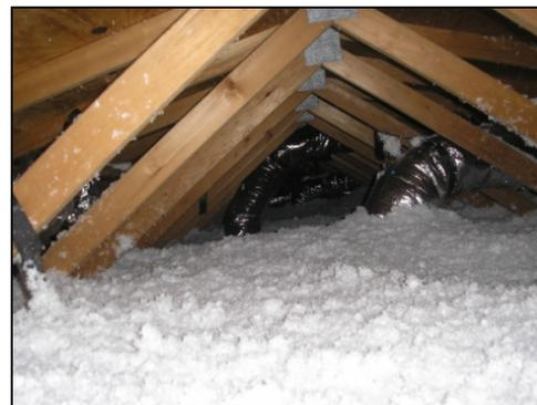
Figure 5 Typical attic insulation pre-retrofit (top) and post-retrofit (bottom)
