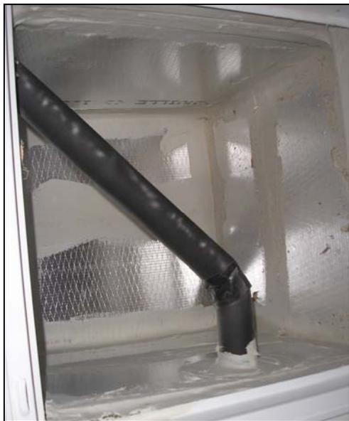
Figure 4 Typical building cavity used as a central return plenum (top) converted to a ducted return sealed with mastic (bottom).
