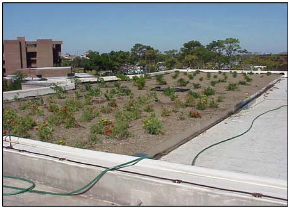
Figure 1. Green roof April 28th, 2005.
