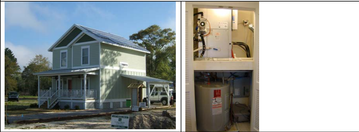
Figure 11. The NZEH by Stalwart Built Homes (l) with its geothermal ht. pump w/ heat recovery DHW (r)
