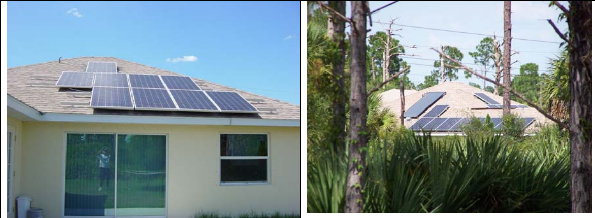
Figure 9. The Schroeders Homes NZEH in North Port, FL. The PV array is split on south and west roofs. Trees shade part of the array and the solar DHW collector in the afternoon
