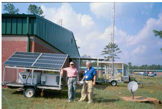
Figure 3: FSEC trailer powering radio station
