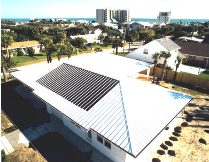
Figure 1. An Example of a BIPV array.
