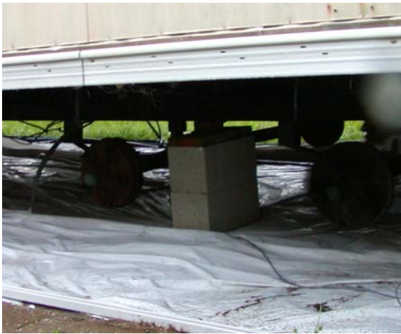
Figure 2 Ground Cover installed
