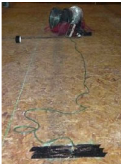
Inline Floor Ducts
