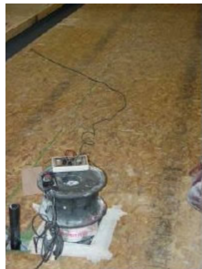
Perimeter Floor Ducts
