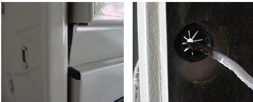
Figure 3 (Left): Example of panel leakage in electric heat AHU. Figure 4 (Right): Thermostat control wire penetration leak area.
