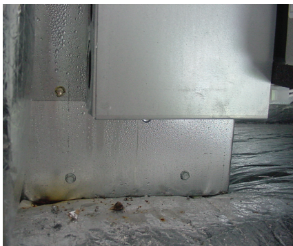
Figure 1: Condensation on metal electric panel inside air handler. Figure 2: Refrigerant line penetration into air handler without seal.
