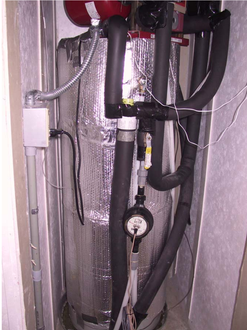
Figure 3 The Solar Hot Water Tank with R5 Insulating Blanket and additional Pipe Insulation Located in the Energy Efficient Manufactured Housing Unit
