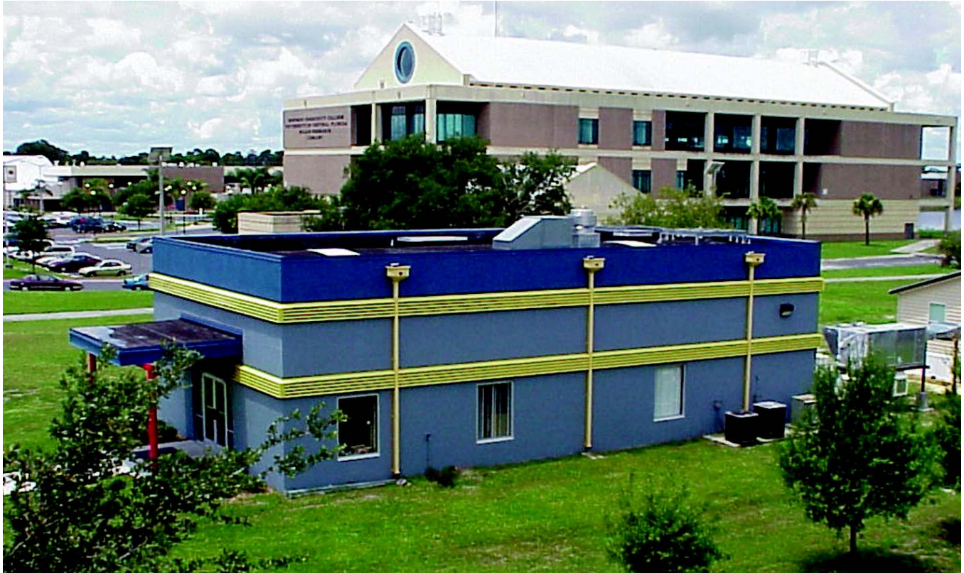
The Florida Solar Energy Center's Building Science Laboratory, site of the field test of the prototype rooftop unit.
