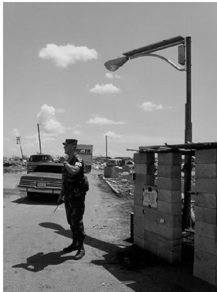
Figure 8. PV Lighting at Security Checkpoint
