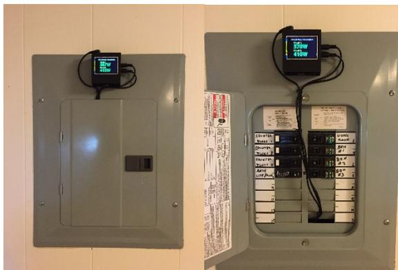
**Figure 3.3:** A SPM meter developed at the University of Hawai'i is installed in the circuit breaker box of a home taking part in the pilot project.
