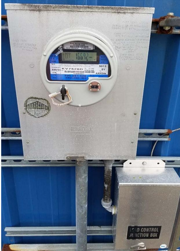
**Figure 1. FSEC Facility Electric Meter and Junction Box Access to Switch Mechanism**
