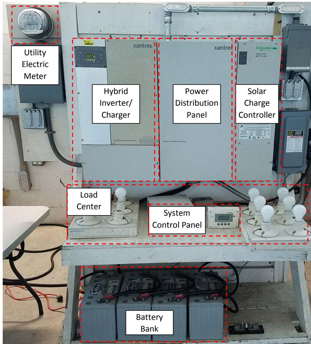
**Figure 6. Photovoltaic Training Panel and Hardware**
