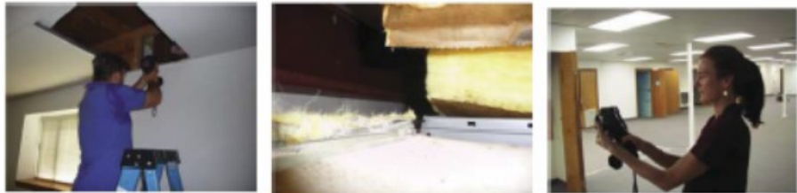
Infrared inspection of insulation – ceiling above acoustic tile drop ceiling
