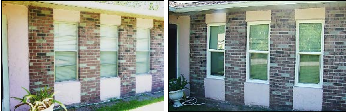
Figure 48. Window retrofit for Site 23: pre-retrofit with existing single-pane, metal-framed windows (left); post-retrofit with double-pane, vinyl-frame windows (right)
