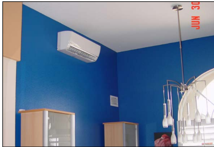
Figure ES-1. Installation of supplemental MSHP at Site 5
