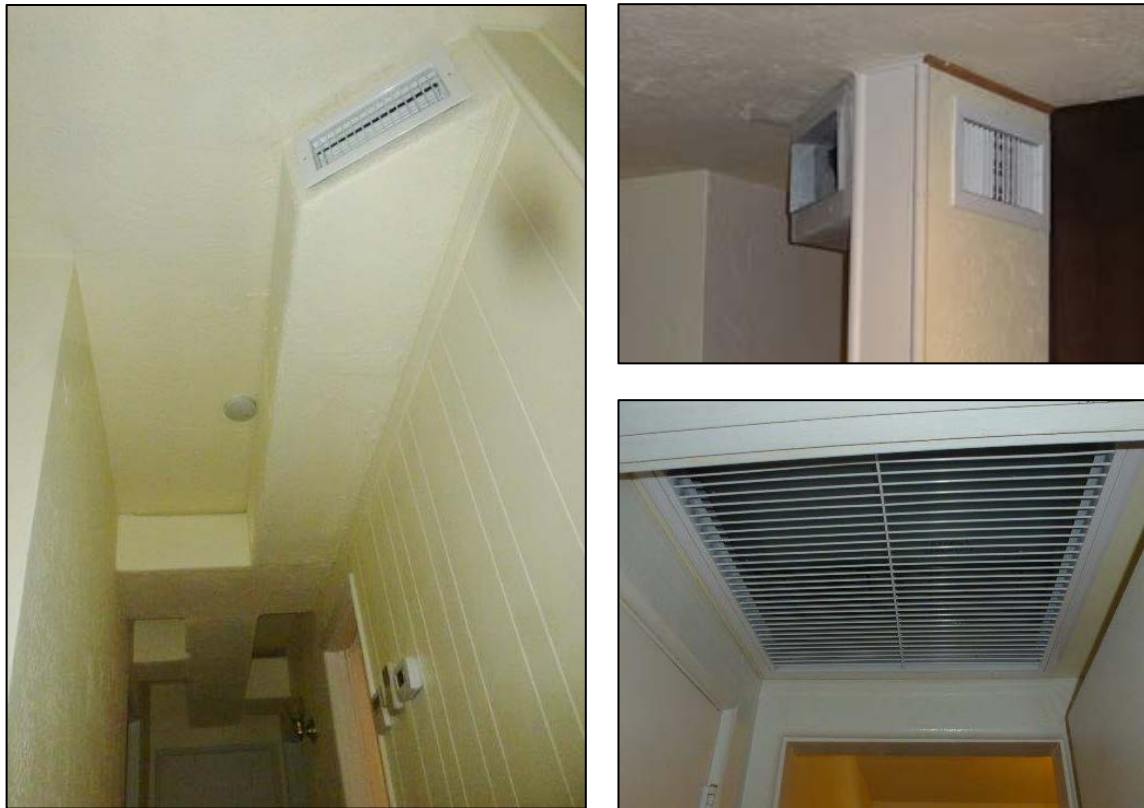
Figure 26. Finished ducted MSHP installation: ductwork (left and upper right) and fan coil (lower right)
