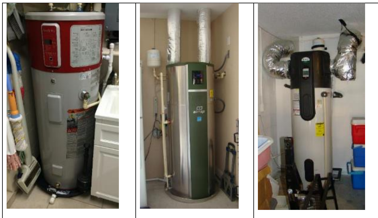
Figure 30. HPWH configurations: interior GE unit in utility room at Site 13 (left); ducted Air Generate unit at Site 5 (center); ducted A.O. Smith unit at Site 26 (right)
