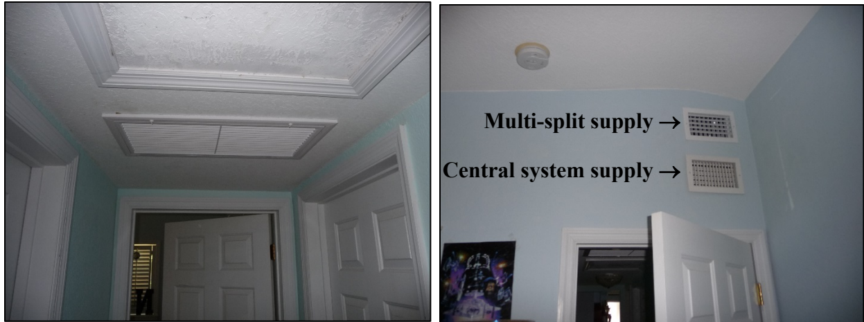
Figure 14. Ceiling-mounted fan coil return grille (left); existing and new supply registers (right)
