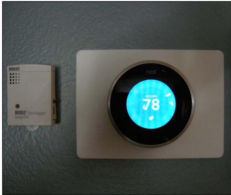
Figure 63. The Nest learning thermostat installed at one of the PDR sites showing the redundant temperature and humidity measurement
