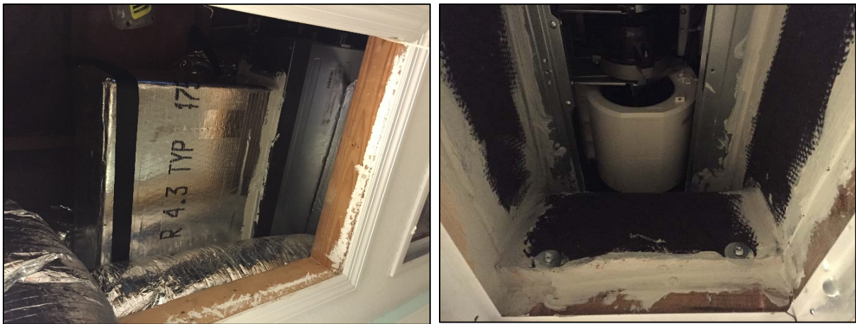
Figure 13. Fabricated junction box installed above attic hatch (left); return plenum and mini-split fan coil installed above ceiling penetration with seams sealed (right)
