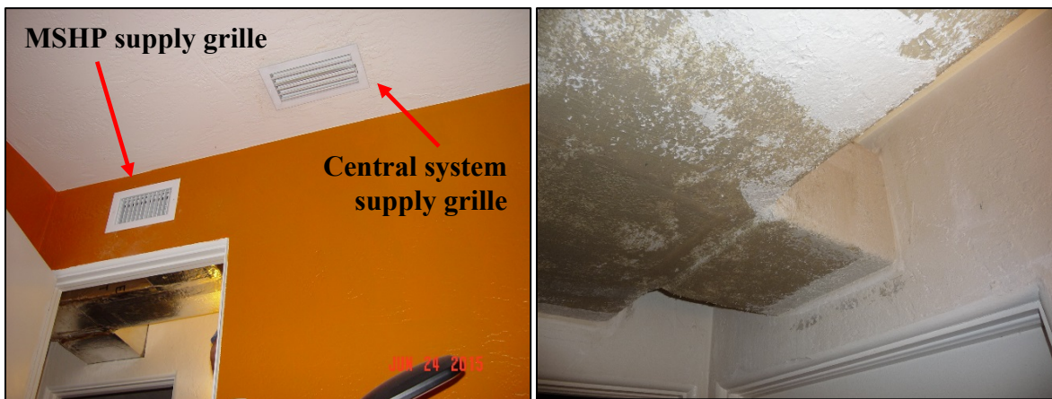
Figure 25. Bedroom view showing both the MSHP and the original central system supply grilles (left); sealed wall penetrations (right)
