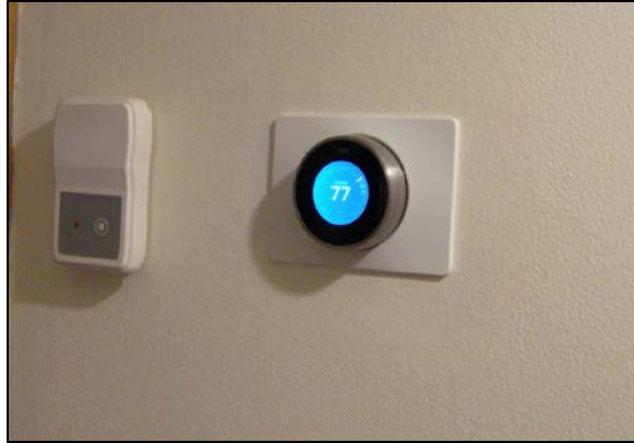
Figure 74. Installed Nest and broadband temperature and RH measurement by thermostat at Site 16
