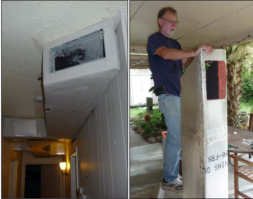
Figure 24. Construction of living room and kitchen supply air duct (left); fabricated ducts installed and sealed with mastic (right)
