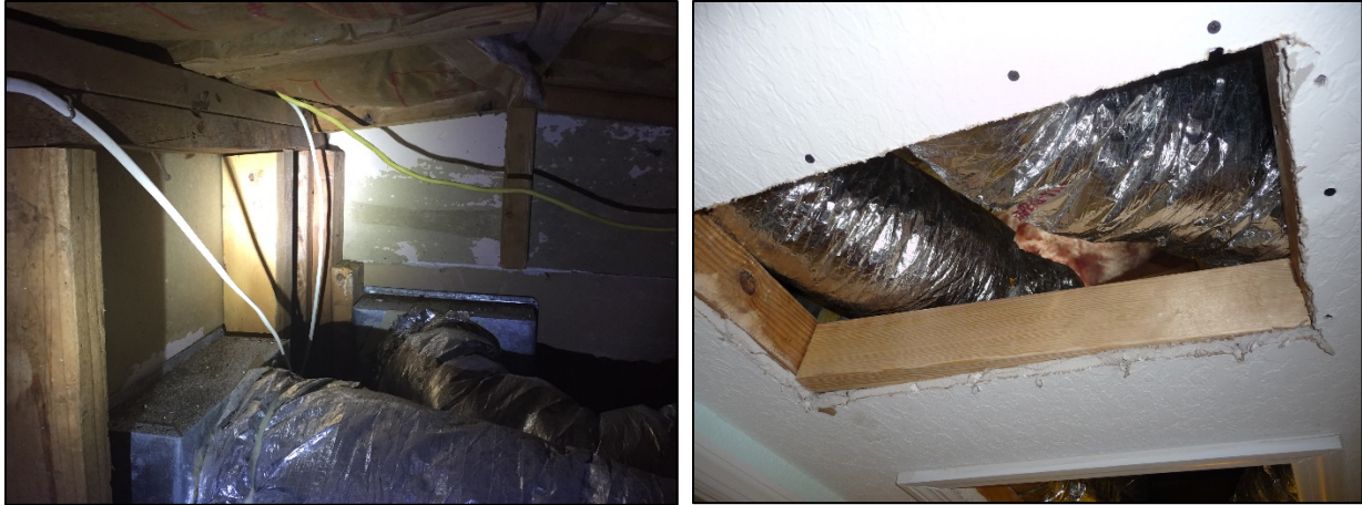
Figure 12. Pre-retrofit attic space used for the ceiling-mounted fan coil and supply air ducting (left); penetration into attic to mount the air handling unit (right)
