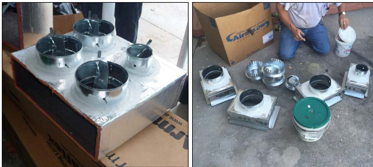
Figure 11. Dampered collars for four supply ducts attached and sealed to fabricated junction box (left); supply register boots sealed with mastic (right)
