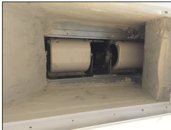
Figure 16. Air barrier applied to inside of return plenum
