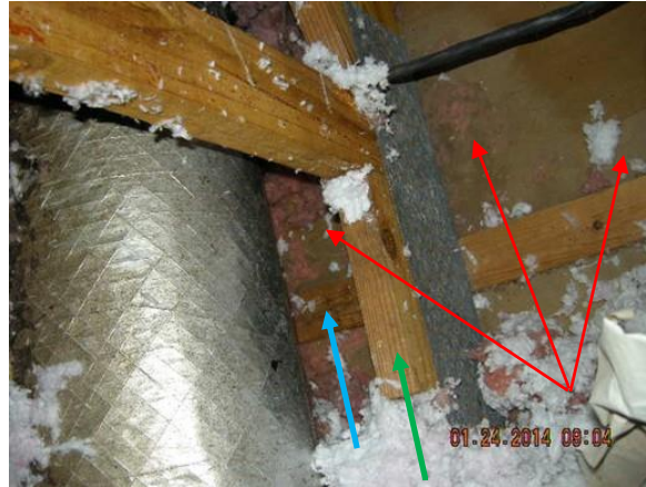
Figure 12. Past water stains observed in ceiling drywall directly above living room
