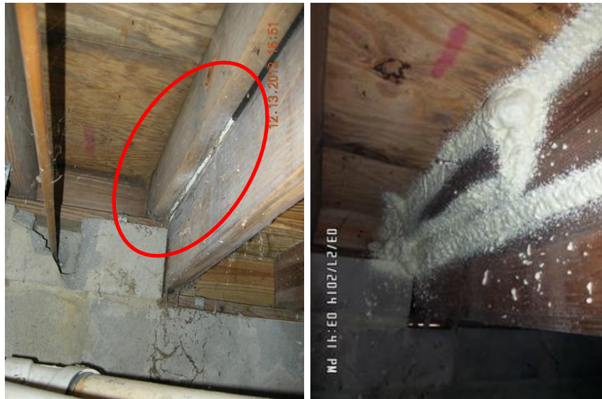
Figure 20. Crawlspace floor transition areas unsealed (left) and sealed (right)
