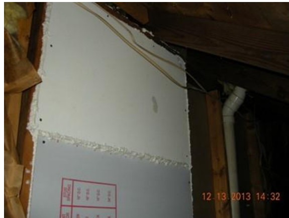
Figure 18. Air barrier installed
