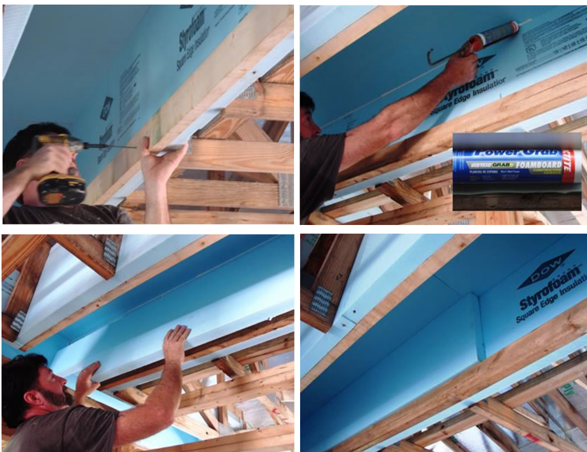
Figure 26. Chace construction overview
