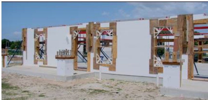
Figure 5. ICF exterior wall under construction
