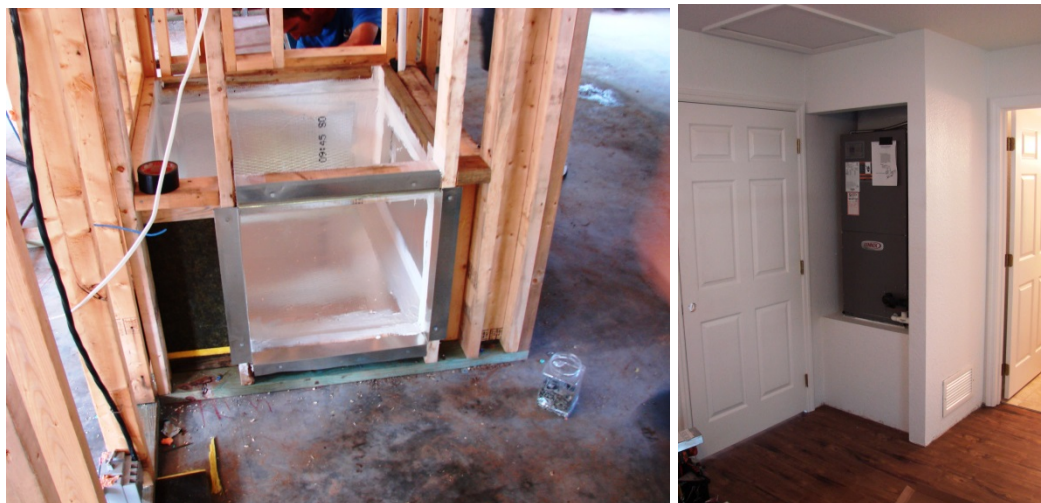
Figure 18. Construction of air handler closet
