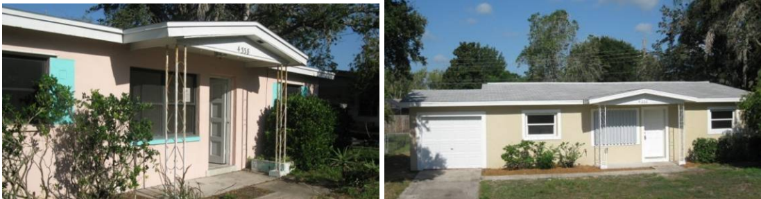
Figures 39-40. EH-07 pre-retrofit (left) and post-retrofit (right).
