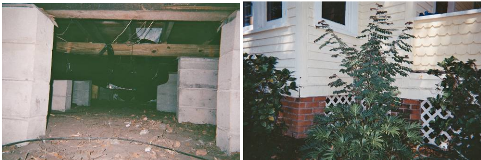
Figures 4-5. EH-01 pier foundation (left) skirted with vinyl lattice panels (right) provide excellent venting of the open crawl space.
