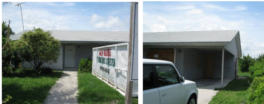
Figures 85-86. EH-20 pre-retrofit
