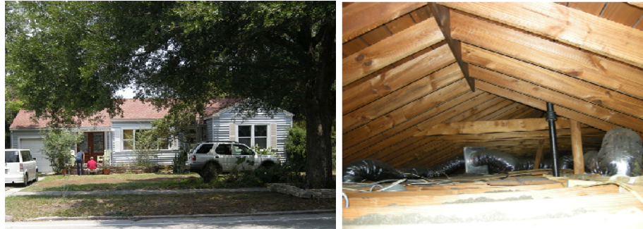
Figures 56-57. EH-15. As found home (left). Attic insulation, head room, and roof framing (right).
