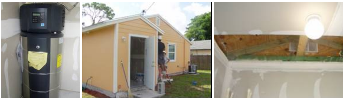
Figures 122-124. The heat pump water heater, HPWH (left) is located inside a small unconditioned room (center) which is connected to the hot attic (right) to provide adequate free air for the proper operation of the HPWH.
