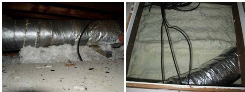
Figures 53-54. EH-14. Old duct work with blown-in ceiling insulation pre-retrofit (Left Photo). Looking up at insulated roof deck with new ductwork inspected prior to hanging sheetrock ceiling (Right photo).
