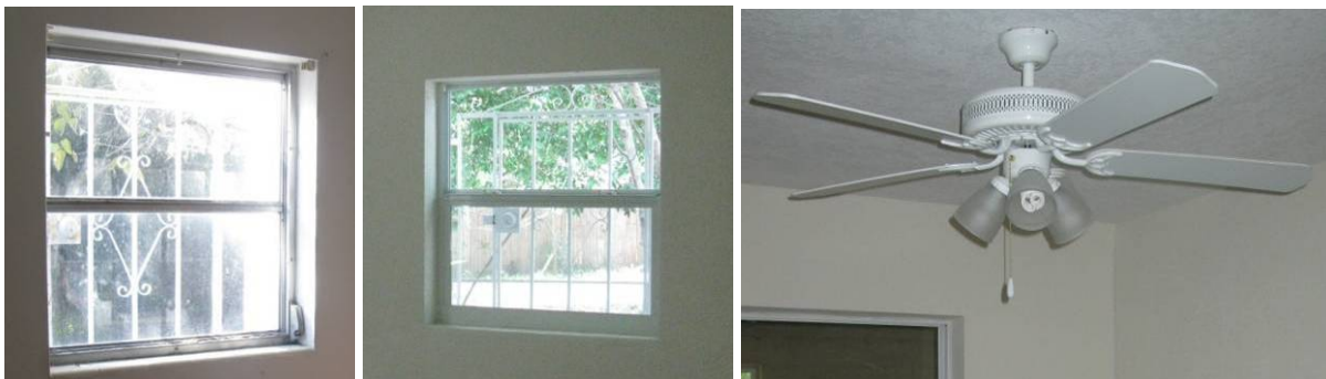
Figures 10-12. EH-02 pre-retrofit awning window (left), post-retrofit Low-E (center), post-retrofit fan with compact fluorescent light bulbs (CFLs) (right).
