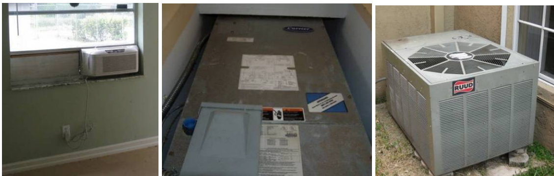
Figures 93-95. Retrofit EH-21 pre-retrofit wall unit (left), Pre-retrofit condenser (center), pre-retrofit air handler (right)
