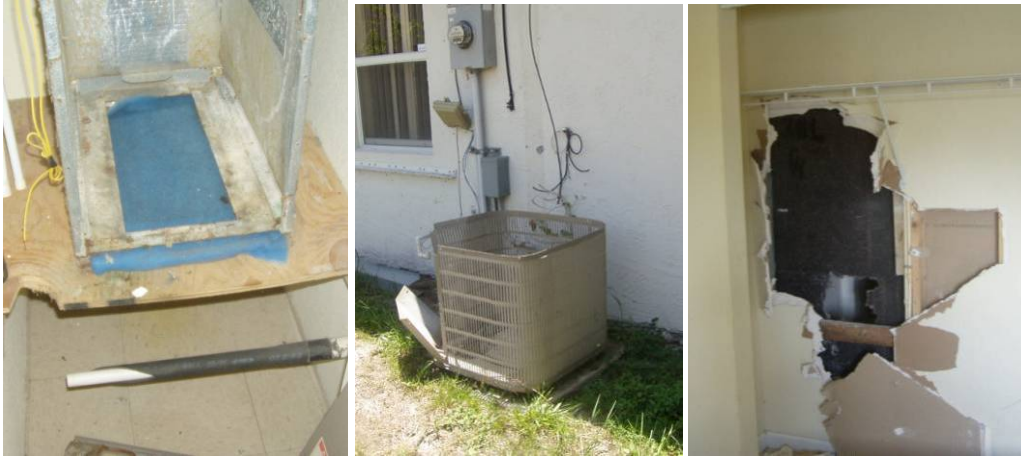
Figures 76-78. EH-19 pre-retrofit air handler (left), compressor (center), interior wall destruction (right)
