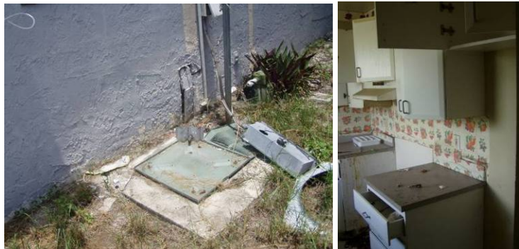
Figures 87-88. Retrofit EH-20 pre-retrofit sight of missing compressor (left), pre-retrofit kitchen missing appliances (right)
