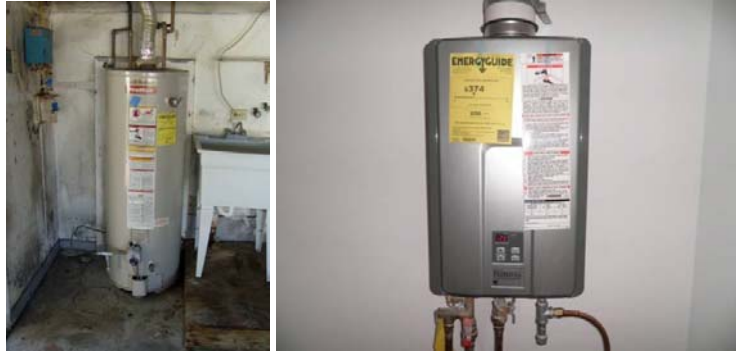
Figures 51-52. EH-14. Switching from an exterior located gas hot water tank (left photo) to an interior mounted instantaneous tank reduced the HERS Index by 7 points and saved an estimated $491/yr in energy use.
