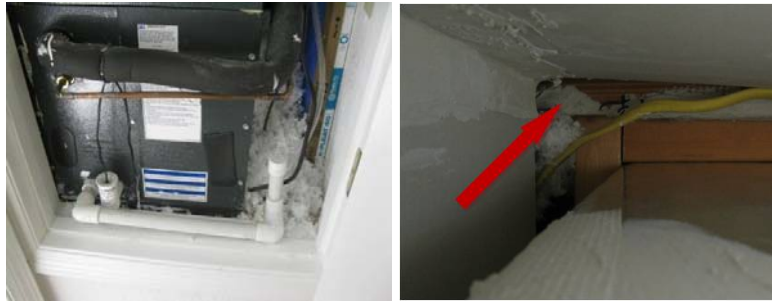
Figures 41-42. EH-07. White attic insulation around air handler (left) fell through spaces in the closet ceiling (right, looking up at closet ceiling framing).
