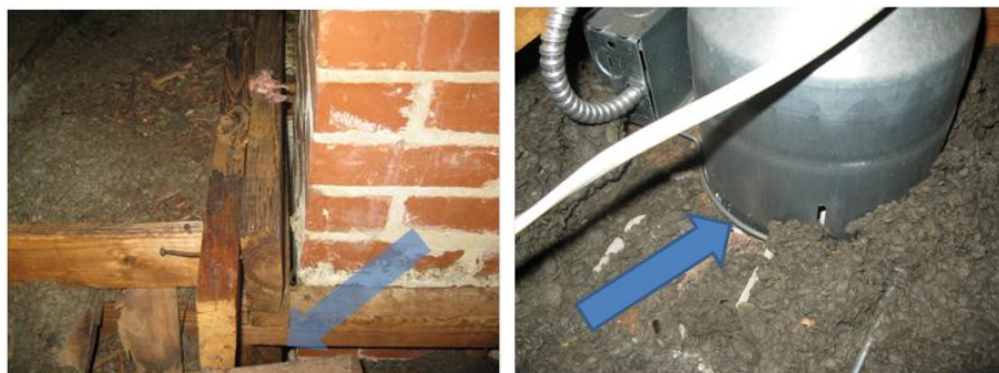
Figures 58-59. EH-15. Air flow pathway from the attic into conditioned space along the fireplace wall (left) and through and around numerous recessed lighting fixtures (right).
