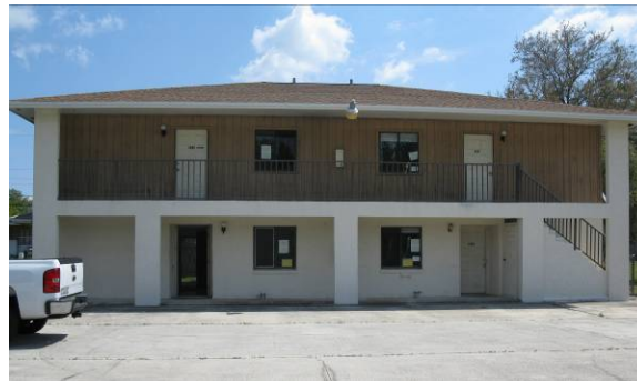
Figure 44. EH-08-11 pre-retrofit, renovation is still in progress
