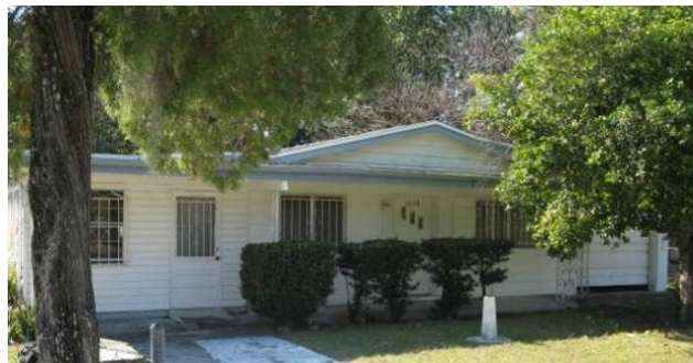
Figure 6. EH-02 pre-retrofit (Post-retrofit exterior unchanged)
