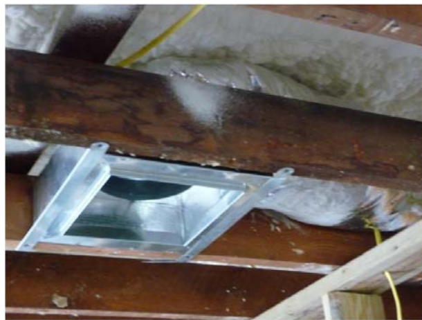
Figure 55. EH-14. A very shallow unvented attic with foam insulation at roof deck resulting in duct compression and an area of thinner insulation.
