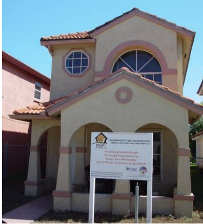
Figure 92. EH-21 post-retrofit (exterior unchanged between pre-retrofit and post-retrofit)
