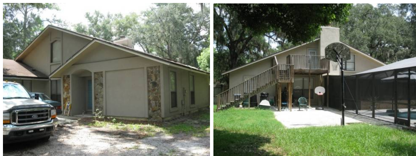
Figures 108-109. EH-23 pre-retrofit
