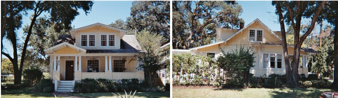
Figures 2-3. EH-01 front (east) and side (south) facades of Craftsman style retrofit candidate.
