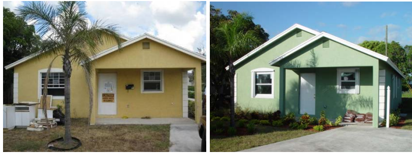
Figure 101-102. EH-22 pre-retrofit (left) and post-retrofit (right)
