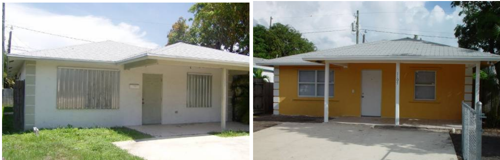
Figures 74-75. EH-19 pre-retrofit (left) and post-retrofit (right)
