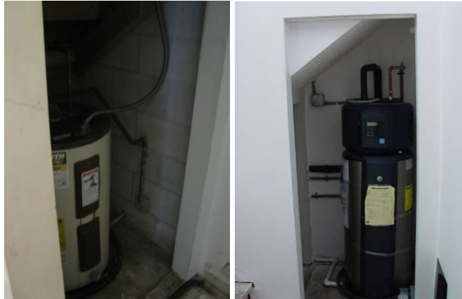
Figures 96-97. EH-21 pre-retrofit electric tank water heater (left), post-retrofit electric hybrid water heater with heat pump (right)
