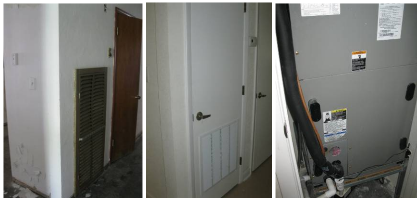
Figures 13-15. EH-02 pre-retrofit abandoned heater (left), post-retrofit closet (center), post-retrofit open return with airflow-restricted louvered doors (right)
