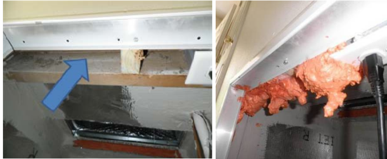
Figures 29-30. EH-04. An open wall cavity connecting the return plenum to the attic was discovered during the test out (left photo with arrow marking air pathway). The opening was sealed using a combination of fiberglass (filler) and expandable foam sealant/insulation (photo right). The excess foam was trimmed before reinstalling the air handler filter and grille.
