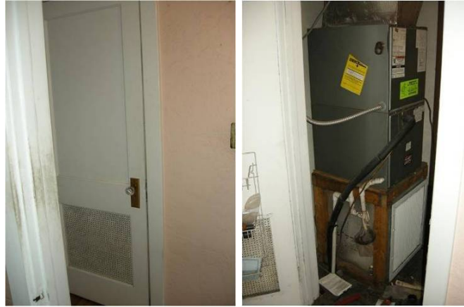
Figures 60-61. EH-15. Air handler located in the central hallway has a door with a small perforated panel for return air (left). Inside the closet (right) is a filter back grille connected to a small return air duct below an up-flow air handler.
