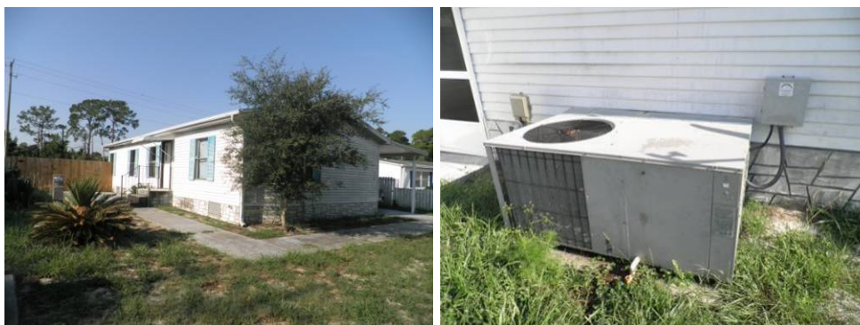
Figures 110-111. EH-24 pre-retrofit manufactured home (left) with central, forced air package unit mechanical system
