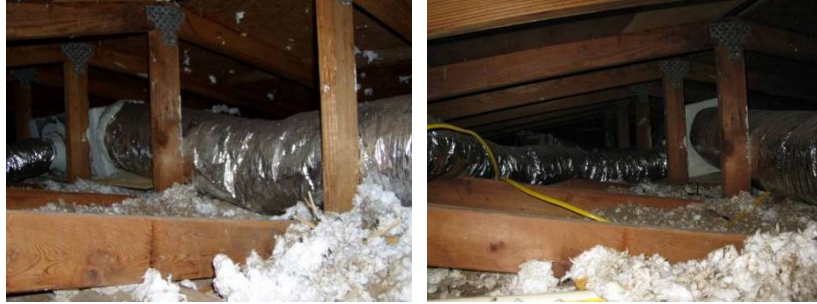
Figures 37-38. EH-06 ceiling insulation: Pre-retrofit estimated average of R-11 (left), post-retrofit no additional insulation (right)
