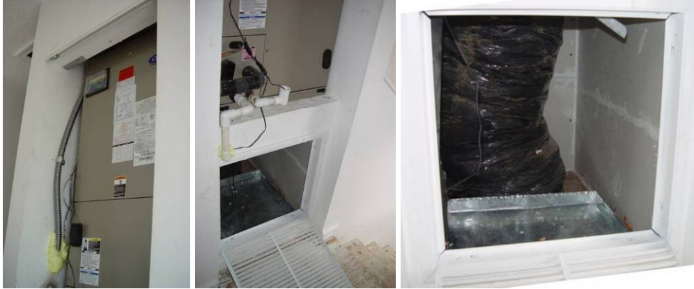
Figures 98-100. EH-21 post-retrofit air handler closet (left), post-retrofit closet (center), post-retrofit open return with airflow-restricted louvered doors (right)
