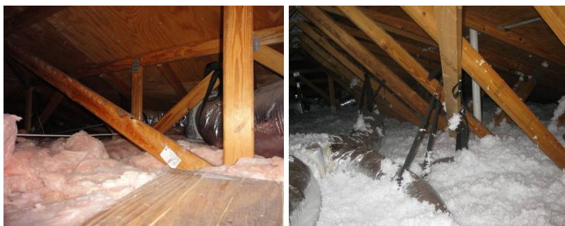
Figures 23-24. EH-03 pre-retrofit (left) and post-retrofit (right) ceiling insulation
