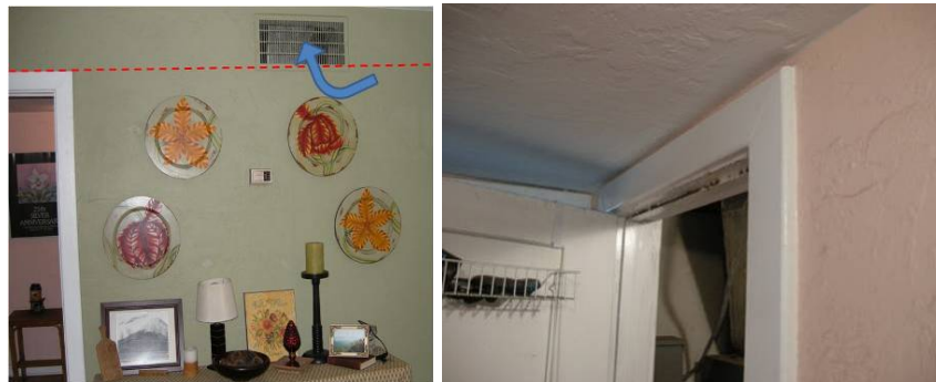
Figures 62-63. EH-15. This wall-mounted passive return air register (left) is connected to a furred down duct chase on the other side of the wall. The bottom of the chase, indicated by the dashed line, forms the ceiling of the adjacent hallway (right).
