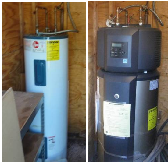
Figures 21-22. EH-03 pre-retrofit electric tank water heater, EF = 0.88 (left), hybrid heat pump water heater, COP = 2.35 (right)
