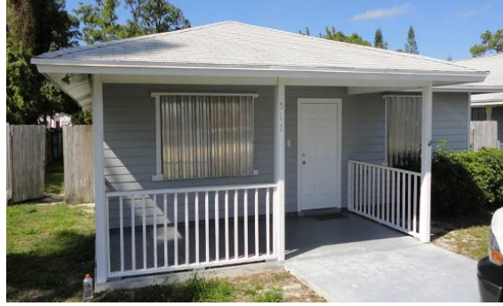
Figure 16. EH-03 pre-retrofit with hurricane shutters in place (Exterior unchanged during retrofit)
