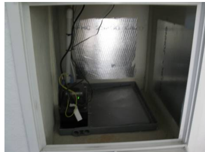
Figure 43. EH-07. New return air plenum constructed of foil faced duct board, shiny side facing in.
