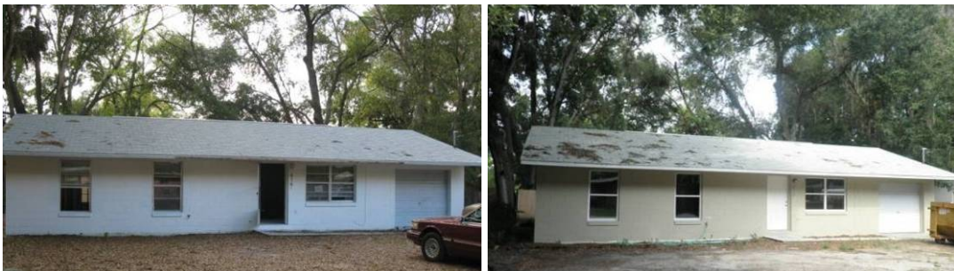
Figures 25-26. EH-04 pre-retrofit (left) and post-retrofit (right)
