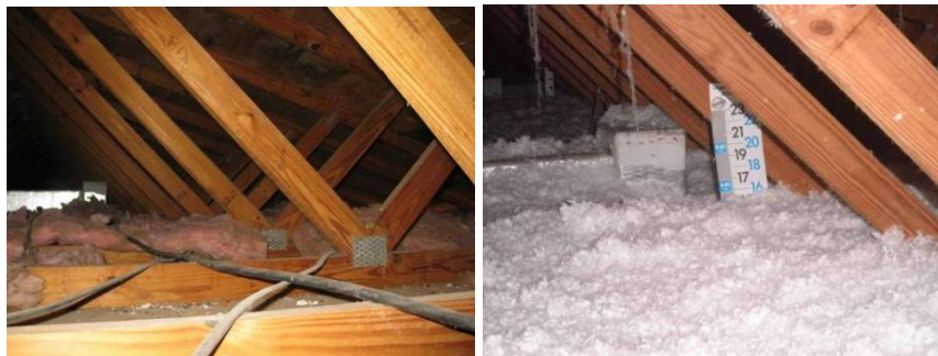
Figures 31-32. EH-04 pre-retrofit compressed fiberglass insulation (left) was improved to R-38 with blown-in fiberglass.
