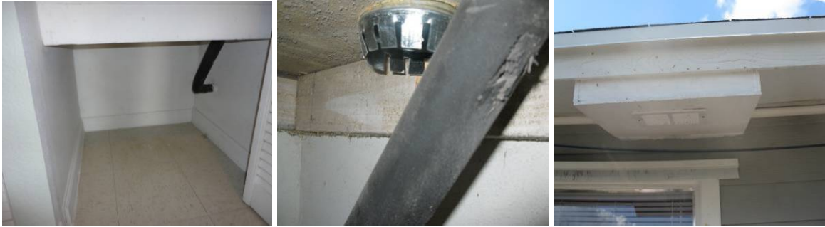
Figures 18-20. EH-03 pre-retrofit return plenum (left), outside air ducted into the post-retrofit return plenum (middle), soffit retrofit for the air intake (right)
