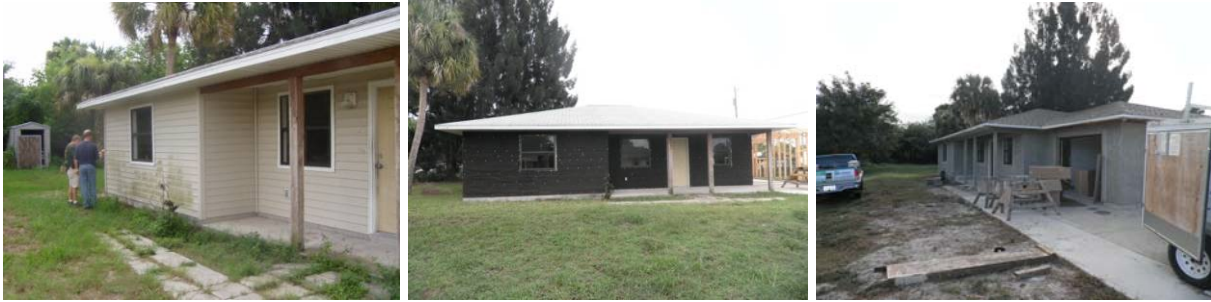
Figures 69-71. EH-17 pre-retrofit (left) midpoint-retrofit (center), December progress (right)
