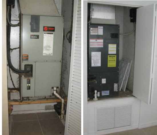
Figures 35-36. Retrofit EH-06. Air Handler Closet: Pre-retrofit without return plenum and installed behind airflow-restricting louvered doors (left), Post-retrofit platform return plenum with filter access on same plane as wall (right).
