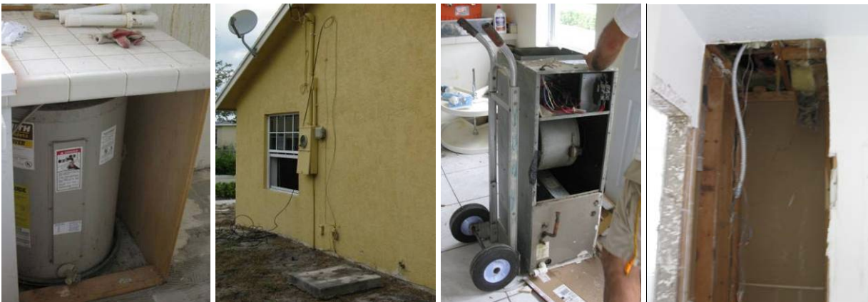
Figures 103-106. EH-22 pre-retrofit water heater (left), missing compressor (center left), dismantled air handler (center right), air handler closet (right)
