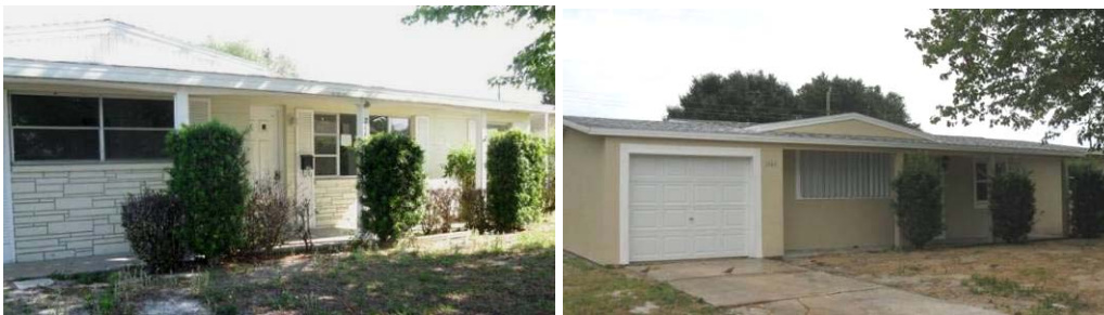
Figures 33-34. EH-06 pre-retrofit (left) and post-retrofit (right).
