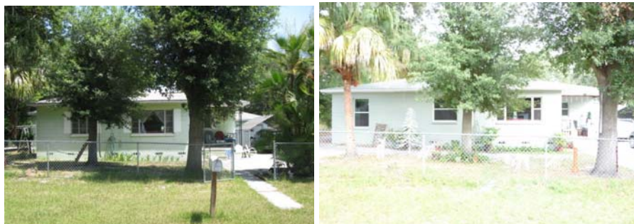
Figures 45-46. EH-12 pre-retrofit and post-retrofit exterior.
