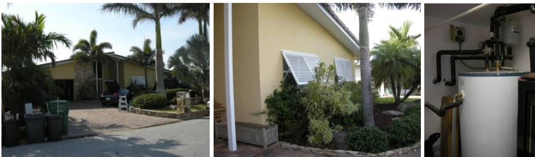
Figures 66-68. EH-16. A number of energy efficiency measures had been incorporated into the home including window shades (middle photo) and a solar hot water system (right photo)
