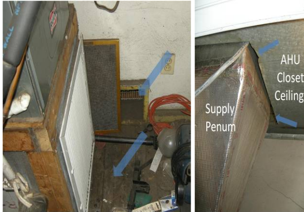
Figures 64-65. EH-15. Uncontrolled air flow pathways in wall and floor (left) and ceiling (of closet surrounding return air plenum).
