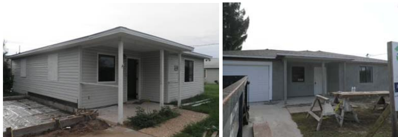
Figures 72-73. EH-18 pre-retrofit (left) and midpoint-retrofit (right).
