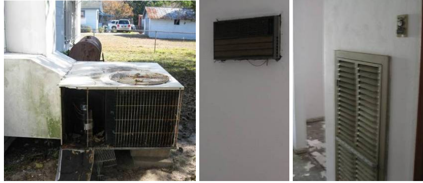
Figures 7-9. EH-02 pre-retrofit package unit (left), wall unit (center), abandoned furnace (right)
