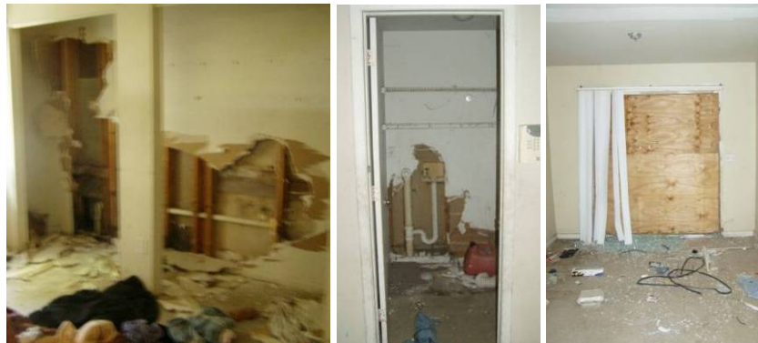
Figures 89-91. EH-20 pre-retrofit vandalized walls (left & center), broken sliding glass door (right)
