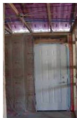
Figure 6-2: RESNET Grade 1 insulation and attic ventilation baffles required for Energy Star certification, East St. Tammany HFH in Slidell, LA
