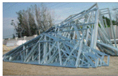
Figure 3-44: Steel trusses produced on site
