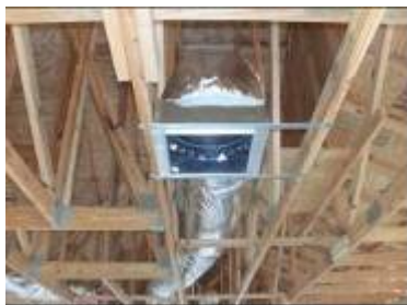
Figure 2-9. Typical new construction ductwork was installed –flexible duct coming from one small fiberglass trunk.
