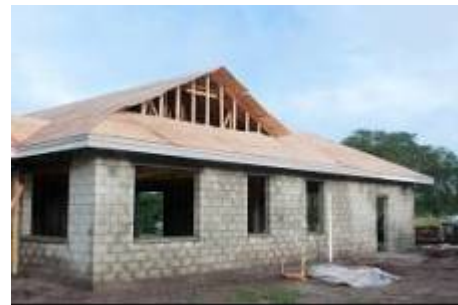
Figure 2-8. September 30 photos shows plywood sheathing near completion. Dutch hip roof design allows for overhang on all four sides while providing an attic ridge area as well.
