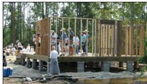
Figure 6-9: Raising Walls at a Gulf Coast Habitat Build
