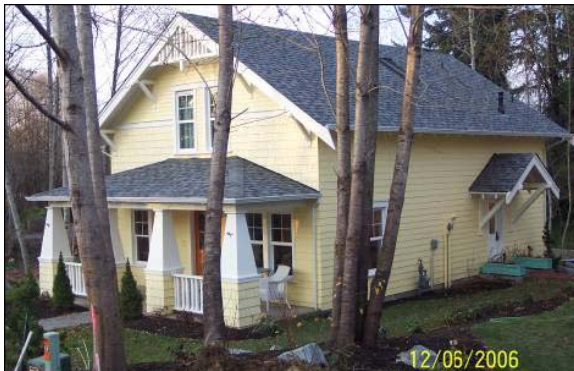
Figure 3-3: Brotherton 13th Ave Bungalows by Scott Homes, Olympia, WA
