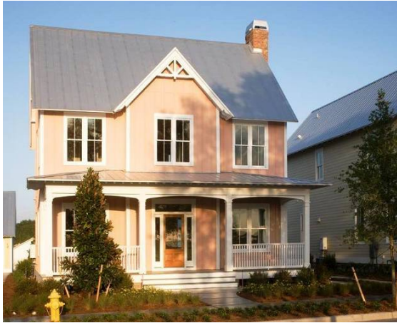
Figure 3-8: Completed Castle & Cooke Home
