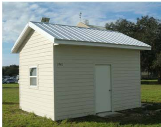
Figure 1- 23: NightCool Shed with White Metal Roof
