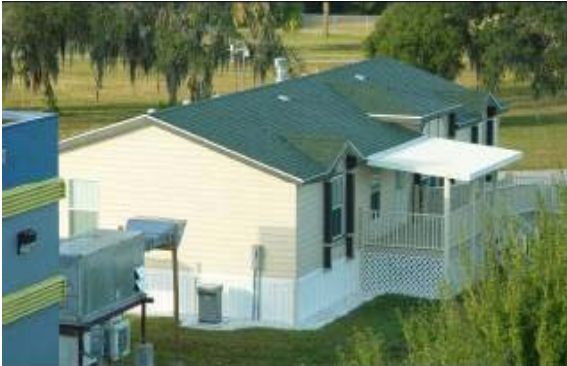
Figure 1- 14: The FSEC Manufactured Housing Lab
