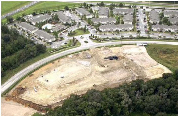
Figure 2-2: Cambridge I Development with Site for Cambridge II Development below.
