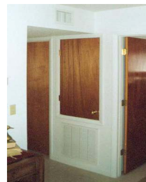
Figure 4-4: An interior air handler, return plenum and supply duct chase
