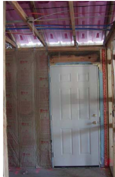
Figure 4-2: RESNET Grade 1 insulation and attic ventilation baffles in High Performance Gulf Coast Affordable Demonstration house built by East St. Tammany HFH in Slidell, LA
