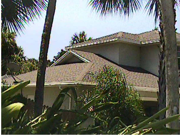
Figure 4-23: East and north side of house with attic over garage adjacent to open floor cavities.
