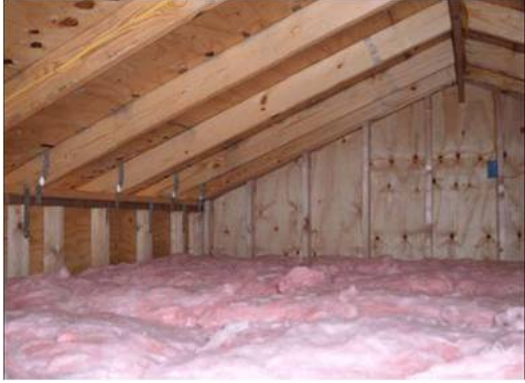
Figure 1- 24: Conventional Shed with Vented Attic and R-30 Fiberglass
