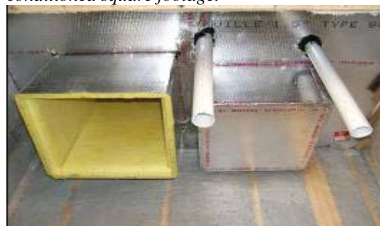
Figure 7: Air barrier in top of air handler closet created with duct board by the mechanical contractor at the time that the ducts are installed.
