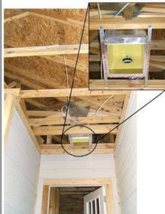
Figure 15 Outside air intake boot in porch ceiling at front door
