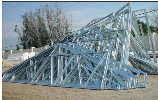
Figure 2-27: Steel trusses produced on site
