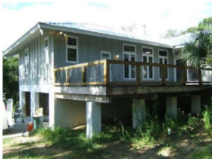
Figure 2-14: Back view of Marquis Construction home in Dade City, FL
