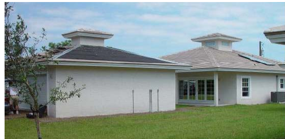
Figure 2-28: Homes with solar hot water and BIPV on detached garage (not installed yet)
