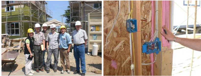
Figure 15 – Rainier Vista development, Habitat for Humanity, Seattle Washington (left), Owens Corning Energy Complete demonstration (right)
