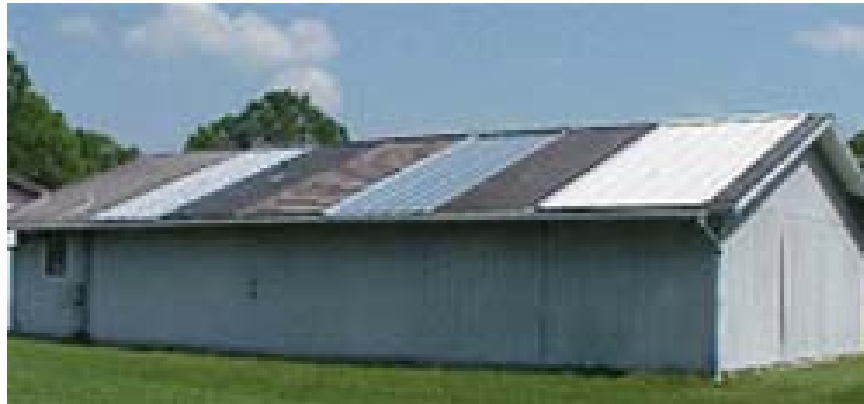
Figure 1-20: The FSEC Flexible Roof Facility (FRF)
