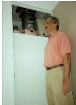
Figure 1-12: Interior view of the Comboflair System with Mr. Henry Delima, Comboflair project director
