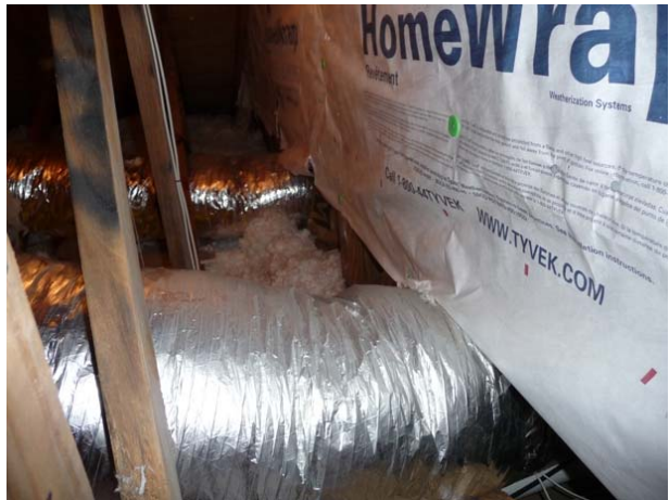
Figure 4-26: Open floor cavity area in the west attic. (west side is to the left)
