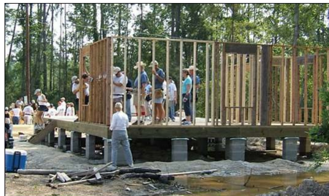
Figure 4-10: Raising Walls at a Gulf Coast Habitat Build
