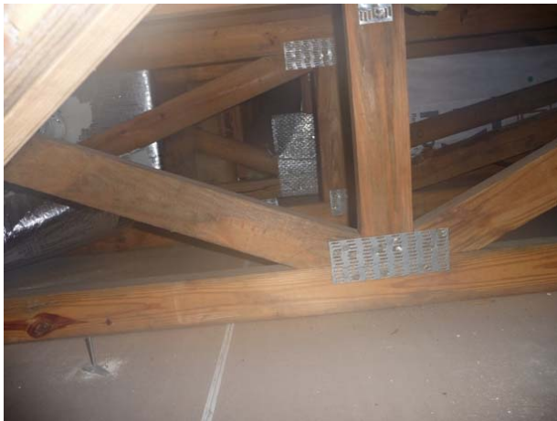
Figure 4-25: Open floor cavity area in the east attic. (view looking toward the west into the floor space)
