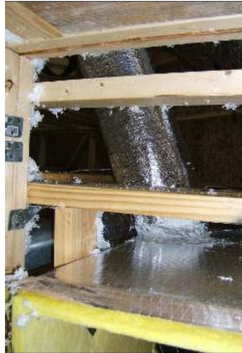
Figure 16 Outside air ventilation duct termination into return plenum
