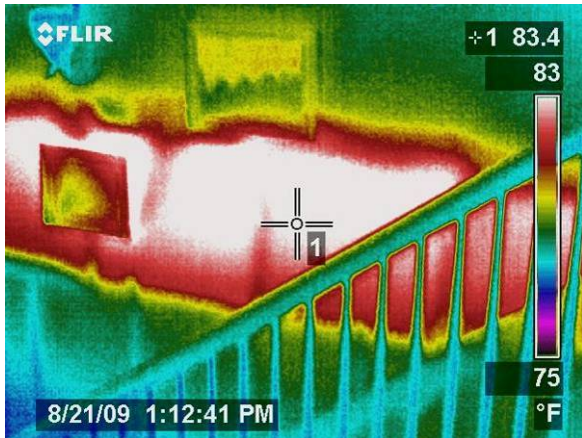
Figure 4-27: Infrared image of floor space behind wall.
