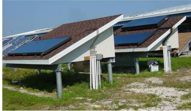
Figure 1-28: The solar collectors are mounted on a nearby roof mock up, with the ICS system in the rear top
