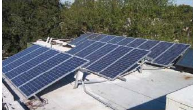
Figure 2-45 2.25kWp Photovoltaic power system on roof top of 2007 TNAH
