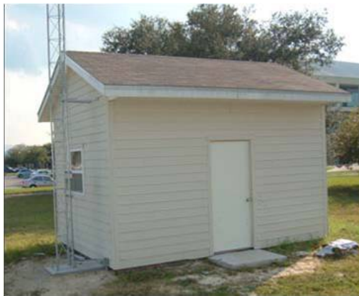
Figure 1- 22: Conventional Shed with Dark Shingle Roof
