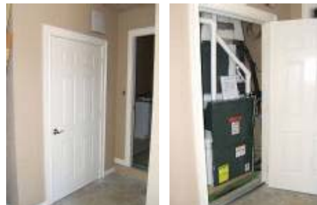
Figure 6: Exterior walls around air handler isolate closet from garage, create valuable conditioned square footage.
