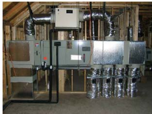
HVAC Equipment Installed
