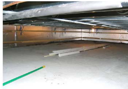
Figure 2-13: Weather tight and insulated crawlspace
