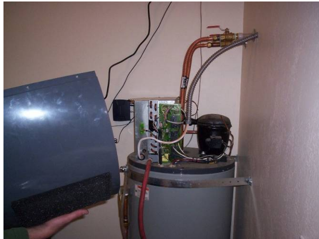
Figure 6a, 6b - Stamets ground source heat pump earth loop charge, and heat pump water heater
