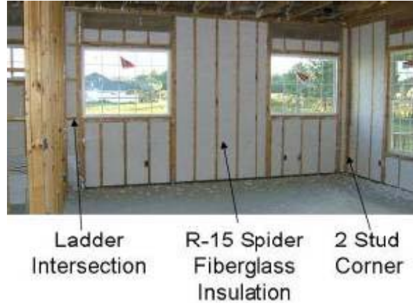
Figure 13 Details reduce framing fraction and improve comfort.
