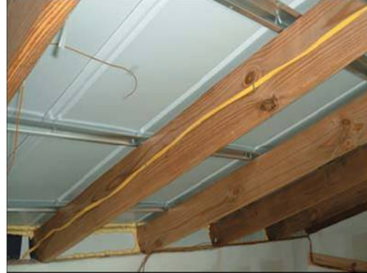
Figure 1- 25: Exposed Metal Roof in NightCool Attic
