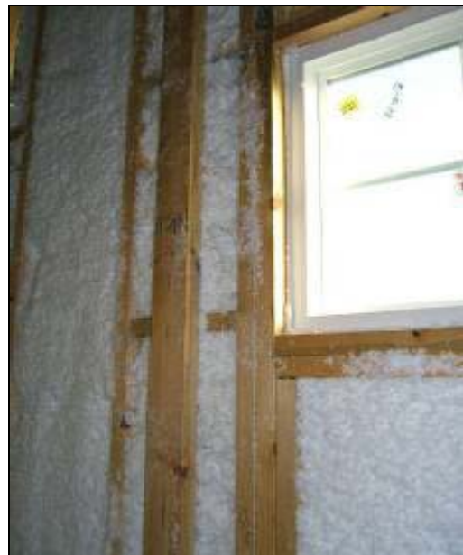
Figure 14 Close up of ladder detail at the intersection of an interior wall. “Rungs” provide drywall nailing surface without compromising insulation.
