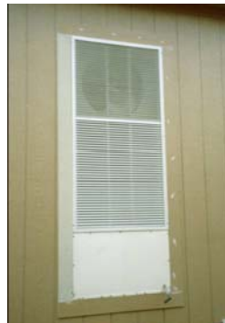
Figure 1-13: Exterior view of the Comboflair under test in Austin, TX at the Palm Harbor Home model center
