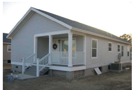
Figure 4-11: Palm Harbor Homes built in Alabama for Oprah Winfrey-HFH partnership
