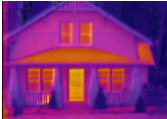
Figure 3-19: Infrared Image of Brotherton 13th Ave Bungalows
