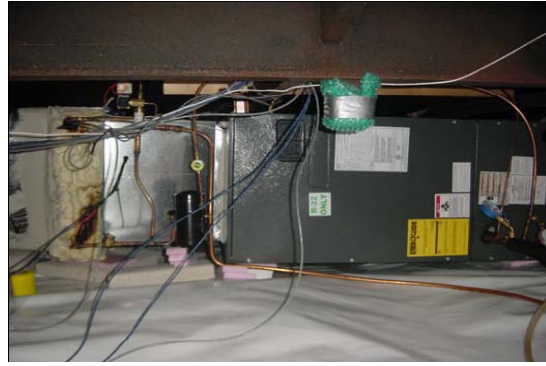
Figure 1- 15: Completed ACDM Indoor unit in the MHLab crawlspace
