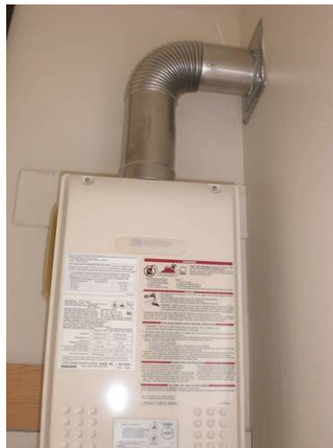
Figure 13 – Noritz tankless water heater – Fort Lewis
