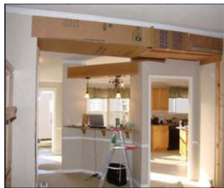
Figure 1-4: Southern Energy Homes Soffit Duct Mockup
