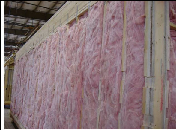
Figure 4. Walls are insulated while the home is still in the factory.
