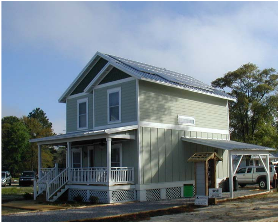
Figure 19. The shadows seen in the photo show the PV modules are partially shaded by a large tree.
