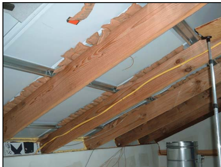
Figure 28. Desiccant paks friction fit between rafters and metal roof.
