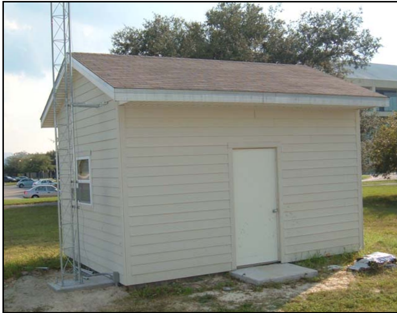
Figure 4. Control test building with conventional asphalt shingle roof covering a ventilated attic.
