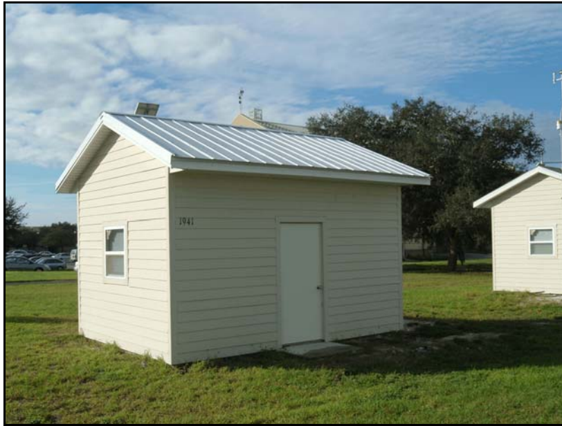
Figure 6. NightCool test building with metal roof.
