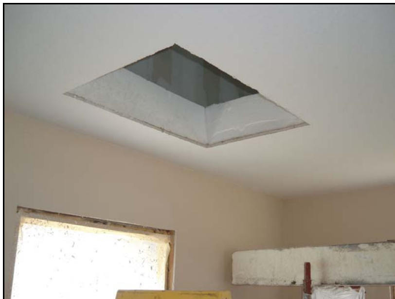
Figure 9. R-30 polystyrene structurally insulated panel (SIPs) ceiling in the experimental NightCool building showing cut-out for attic hatch.
