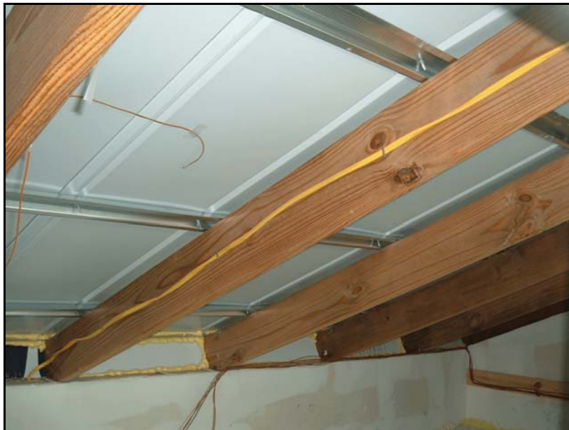
Figure 7. Interior detail of experimental NightCool sealed attic with exposed metal roofing on metal battens. Note thermocouple measuring underside of roof temperature.
