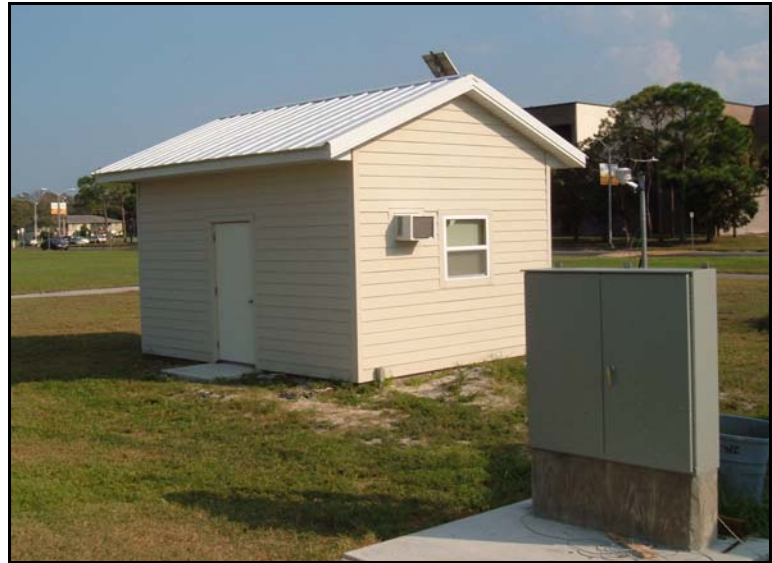
Figure 18. Experimental NightCool building showing central data acquisition system and wall-mounted air conditioner.
