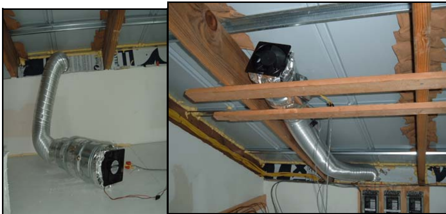
Figure 17. Supply and exhaust attic ventilation fans. These 4-watt fans provide 40 cfm of balanced supply and exhaust air flow when the absolute humidity ratio outdoors is less than that inside the attic space.
