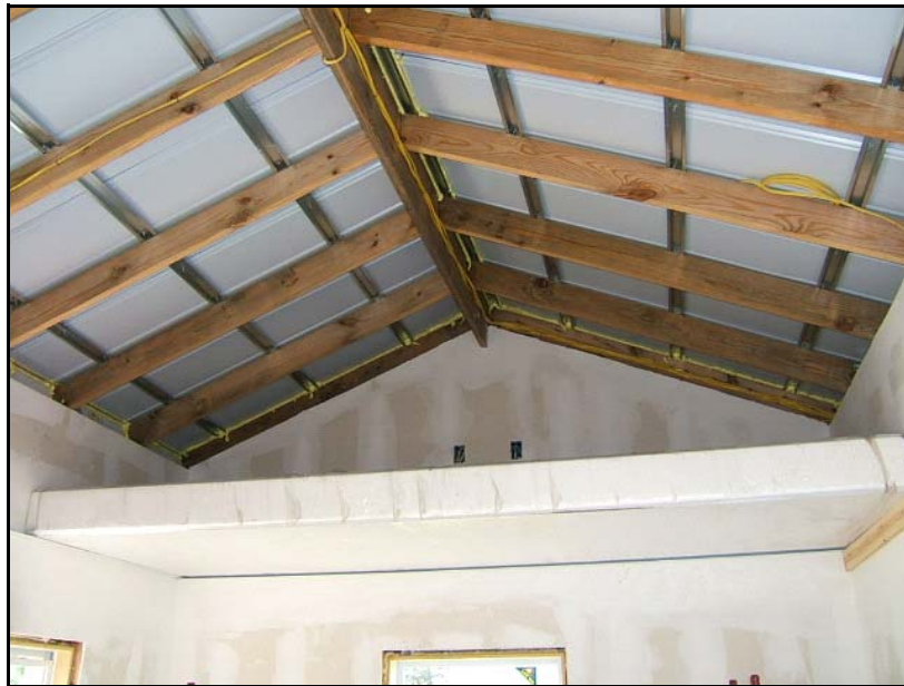
Figure 8. R-30 SIPs panels during installation in the ceiling in the NightCool experimental facility.
