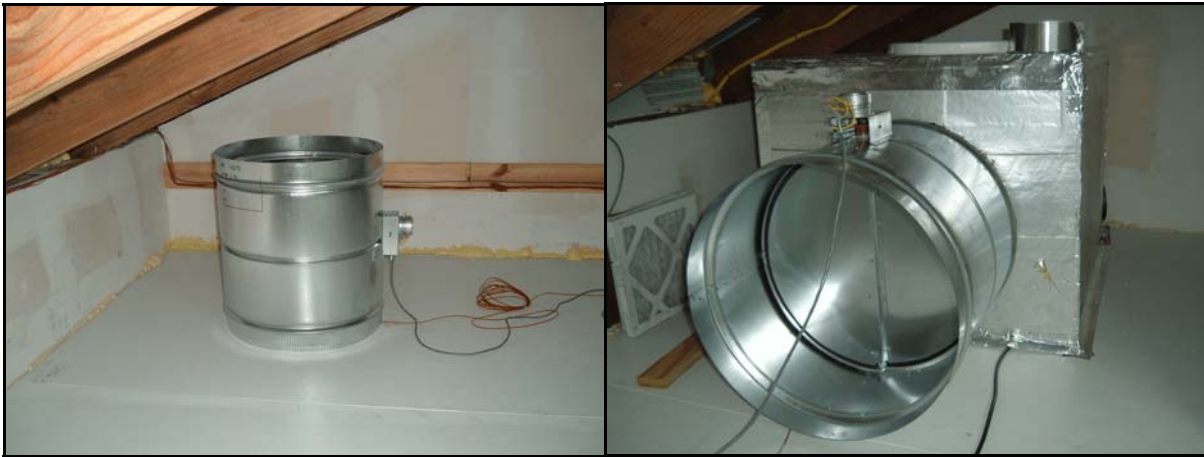
Figure 16. Return and supply side motorized dampers. These close air circulation to the attic when the attic temperature is higher than the main zone.
