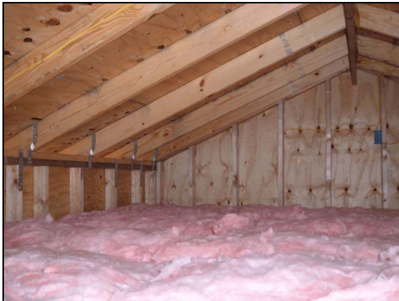
Figure 5. Interior of ventilated control attic with R-30 fiberglass insulation.
