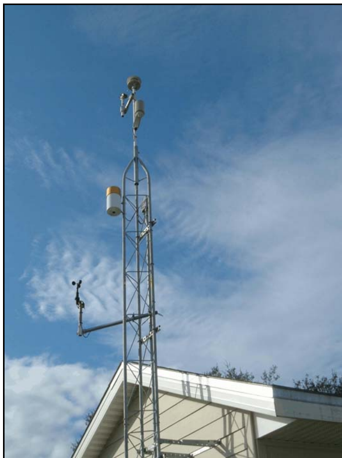
Figure 10. Project weather tower is attached to the control building on the northeast side.
