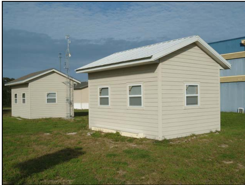
Figure E-1. NightCool side-by-side buildings under test.
