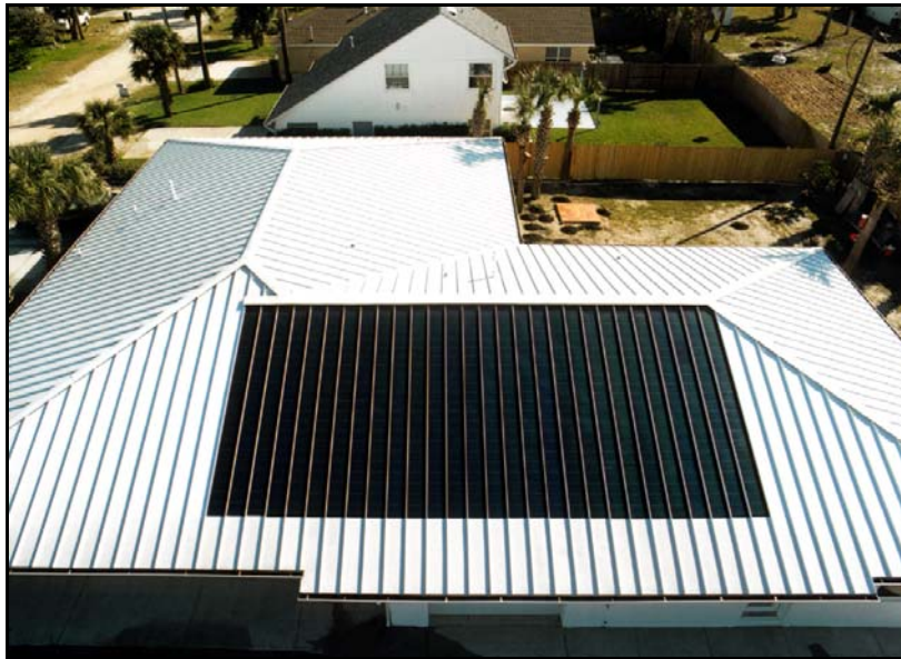
Figure 32. Thin film PV is applied directly to the standing seam metal roof.
