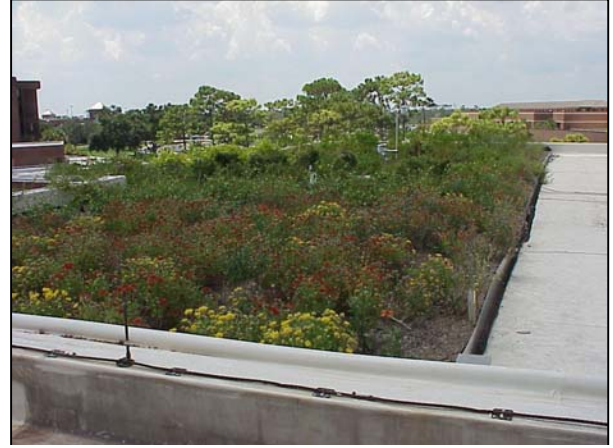
Figure 22. Green roof August 18th, 2005
