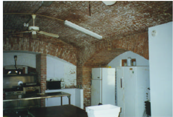
Figure 16. Interior of Crew #4 quarters, showing refrigerators and masonry ceiling.
