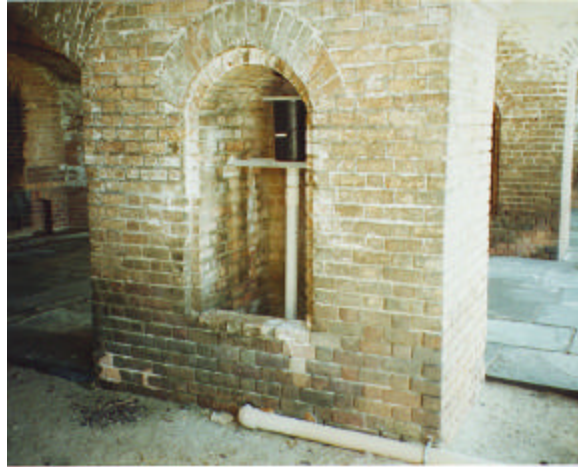
Figure 10. One of original ducts used for rainwater collection.
