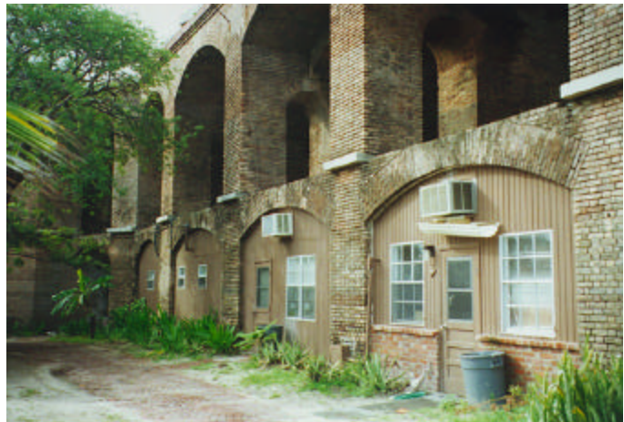
Figure 15. Crews #4 quarters with typical window A/C units.
