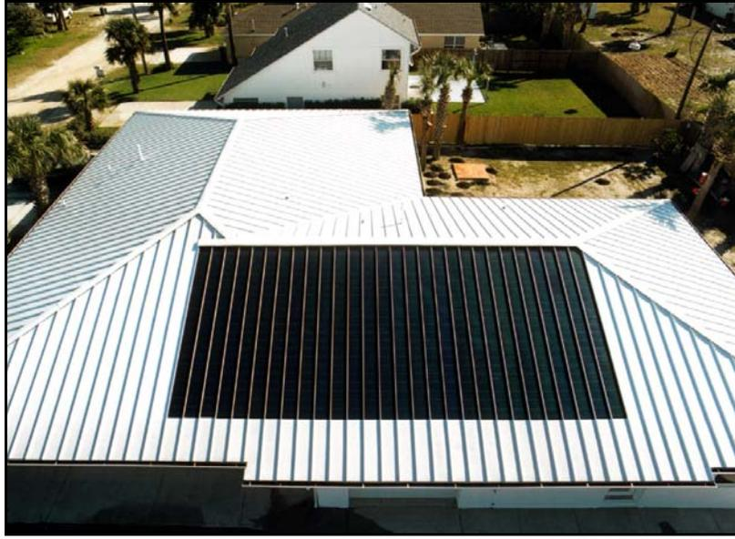
**Figure 31.** Thin film PV is applied directly to the standing seam metal roof.
