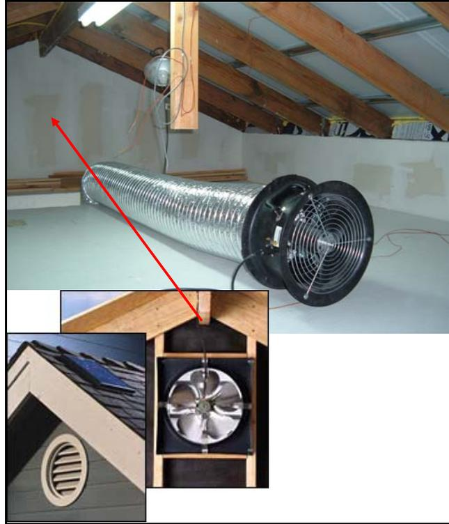
Figure 27. Desiccant dehumidification scheme with solar-powered gable end fans, operated during the day.
