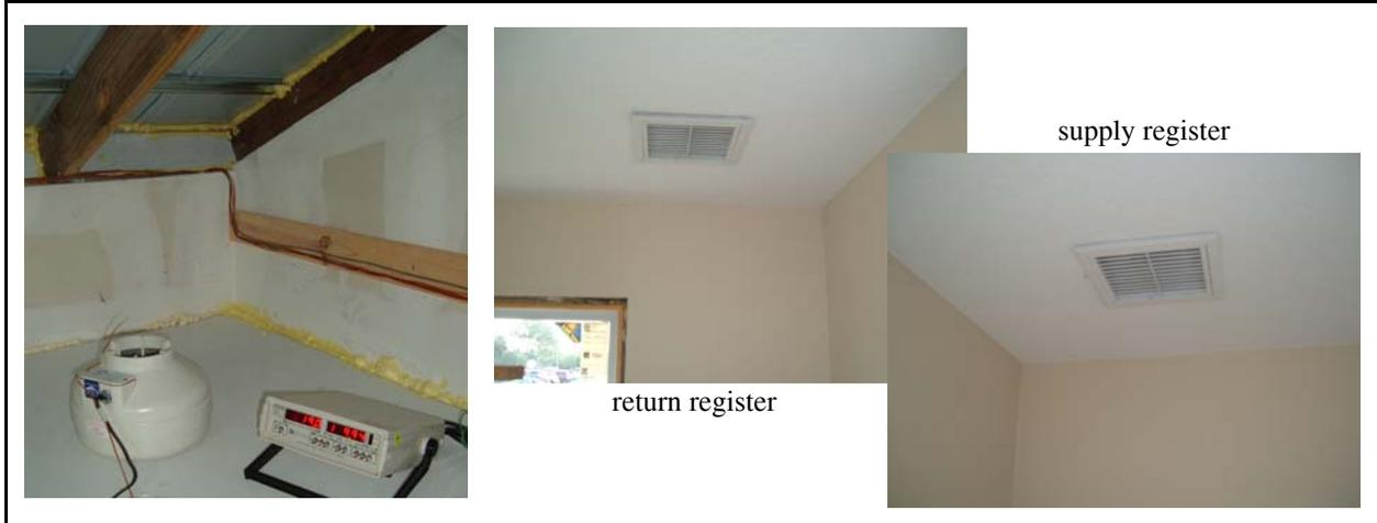
**Figure 14.** High efficiency 150 cfm centrifugal fan and supply and return registers; the current arrangement uses attic depressurization and main zone positive pressure with a single fan operating; the high efficiency fan draws only 18 Watts when operating at full speed.
