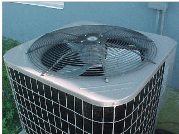
Figure 1. Typical 3-ton (10.6 kW) air conditioner condenser
