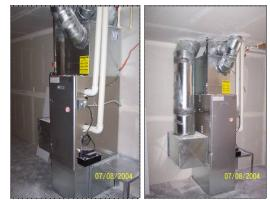
*Figure 46* 90% *AFUE Furnace, as installed at Kokanee Creek*
