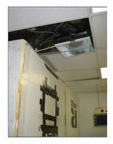
*Figure 110 Return air flow path provided by jumper duct*
