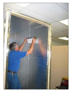
*Figure109* Installing unbaffled return air flow through wall grille
