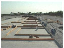
Figure 53 Panel forms on forming bed.
