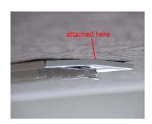
*Figure 95 Gaps at the supply register to drywall joint*
