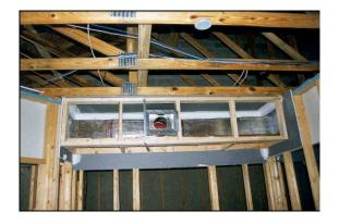
**Figure 41** Interior duct system under construction at Lewis Place – the first Energy Star apartment complex in the country.
