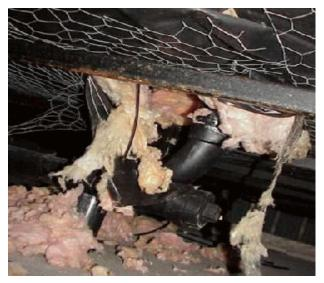
Figure 50 Worst belly tear near plumbing penetration.
