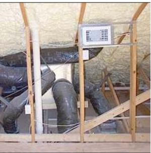
Figure 84 Semi-conditioned space for the ductwork.
