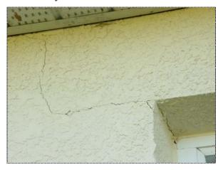
Figure 90 Window corner crack
