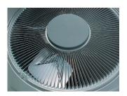
*Figure 97* Air conditioning condenser fan and diffuser.
