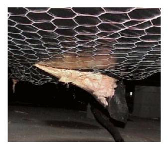
Figure 49 Another belly tear found during inspection.
