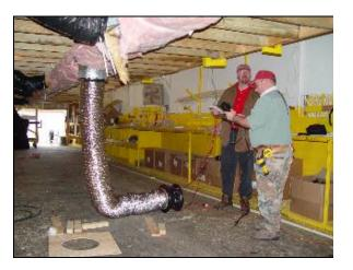
Figure 52 Southern Energy Homes quality control engineer conducts in-plant duct leakage test.
