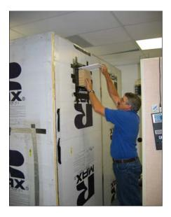
*Figure 108 Installing sound baffled return air flow through wall insert made by Tamarack.*
