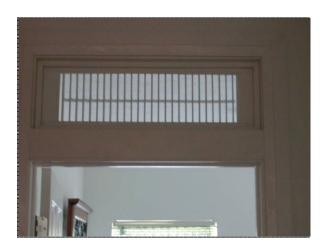
**Figure 28** Transom return air pathway with operable louvers blends in with the vernacular aesthetics of this DESIGNhabitat Energy Star home built in conjunction with Auburn University's College of Architecture.
