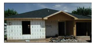
Figure 14 Low income housing built by the City of Lubbock using insulated concrete forms.
