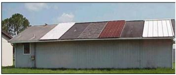
*Figure 106* 2001 *Experimental roof cell. Cells are numbered from left to right starting with the cell second in from the left.*
