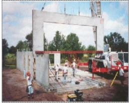
Figure 54 Setting pre-cast concrete wall panel.
