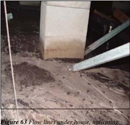
running water under the house. Also note the "tide line" on the support column.
