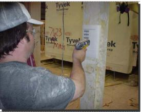
*Figure 51* Scanning *drywall activities with new STACs device.*
