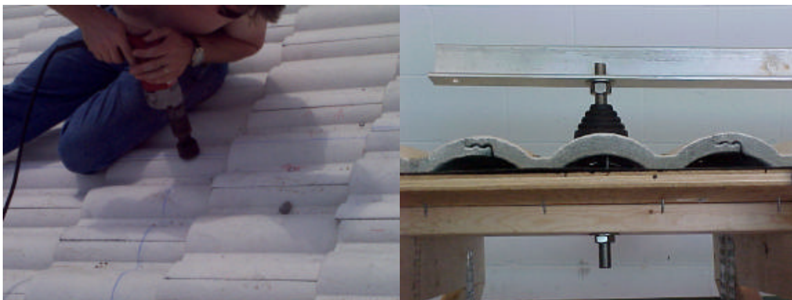
Figures 6a and 6b. A carbide grit hole saw is used to cut through the tile in place and a cross section of the complete assembly.
