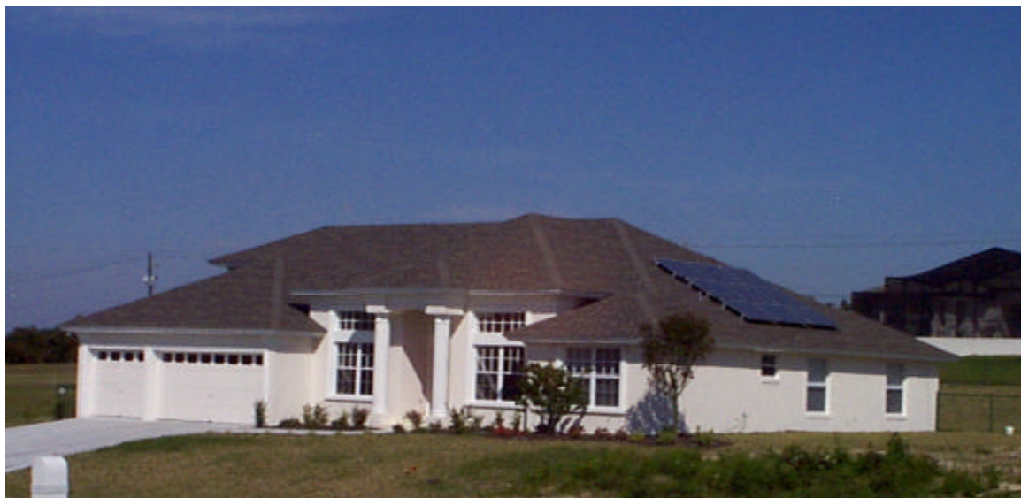
Figure 3. A 2kW utility-interactive system installed on a shingle roof.
