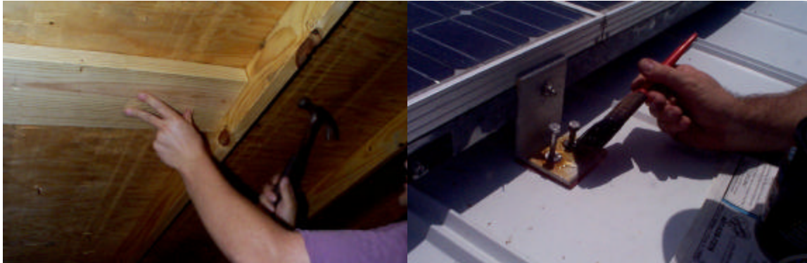
Figures 5a and 5b. Installing blocking between two trusses on the roof deck underside and applying sealant at the penetrations.
