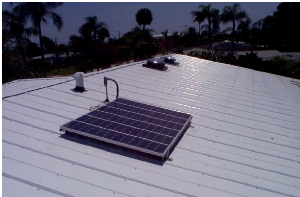
Figure 2. A small standoff mounted PV array installed on a standing seam metal roof.
