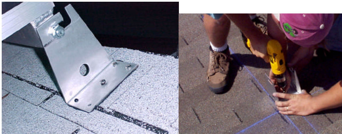
Figures 4a and 4b. A standoff roof mount showing the attachment screw locations and aligning and fastening a roof mount to a shingle roof.
