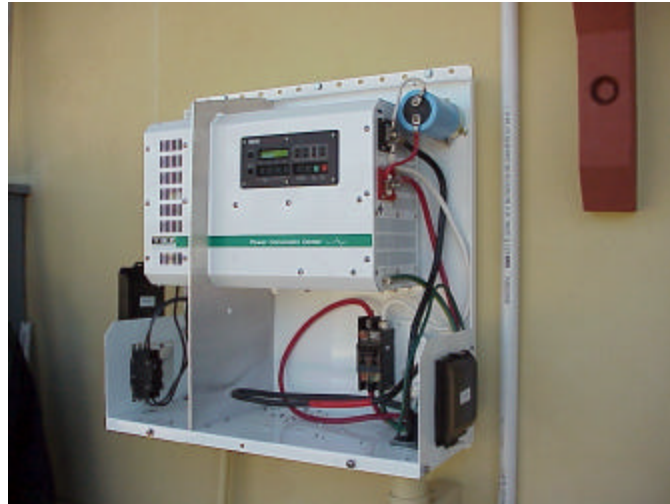
Figure 4. System #1 inverter.
