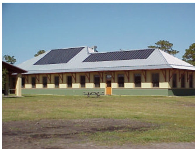
Figure 2. System #1 photovoltaic array.
