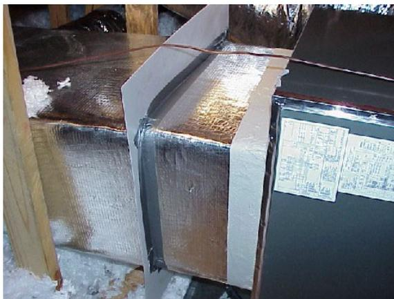
It was not appropriate to cut through the supply plenum in a number of homes, either because there was insufficient space around the plenum, or because the supply plenum was a flex duct. In those cases, the entire duct system was tested. When the entire duct system had to be tested, test pressures were measured in parts of the supply and return ducts as well as in the air handler.
