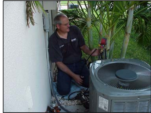
Figure 16. Tune-up and commissioning of new AC system in Merritt Island
