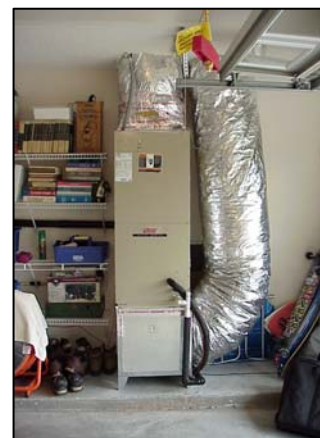
Figure 23. New air handler at Jacksonville site
