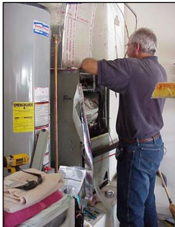
Figure 15. New air handler is installed at the Merritt Island site
