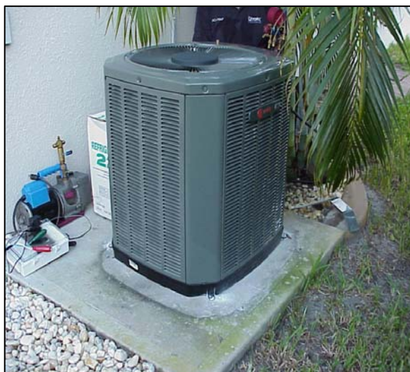
Figure E-1. Outdoor unit of new, properly-sized AC system at Merritt Island house showing footprint of original oversized system on the concrete pad
