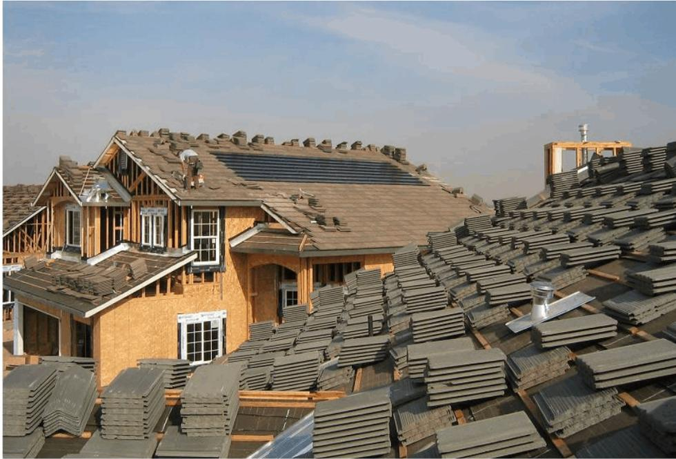
**Figure 4.** Illustration of cross-long width orientation of battens used for installation of tile roof in a California residential development. This arrangement does not provide enhanced ventilation of tile roofing.
