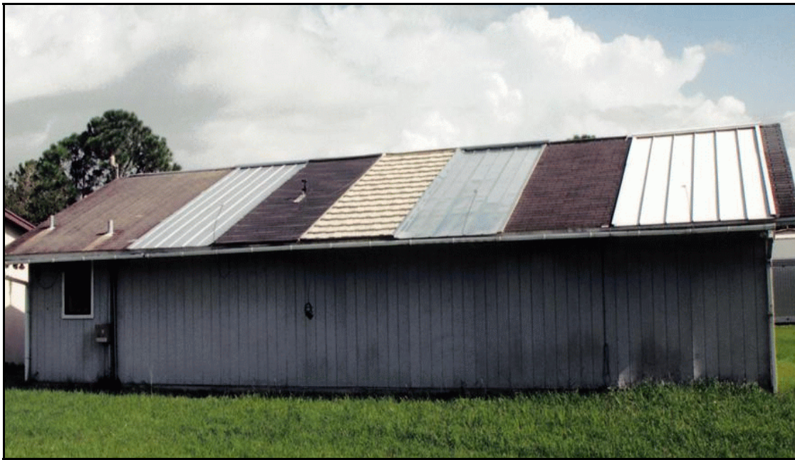
Figure E-1. Flexible Roof Facility in summer 2002 configuration.
