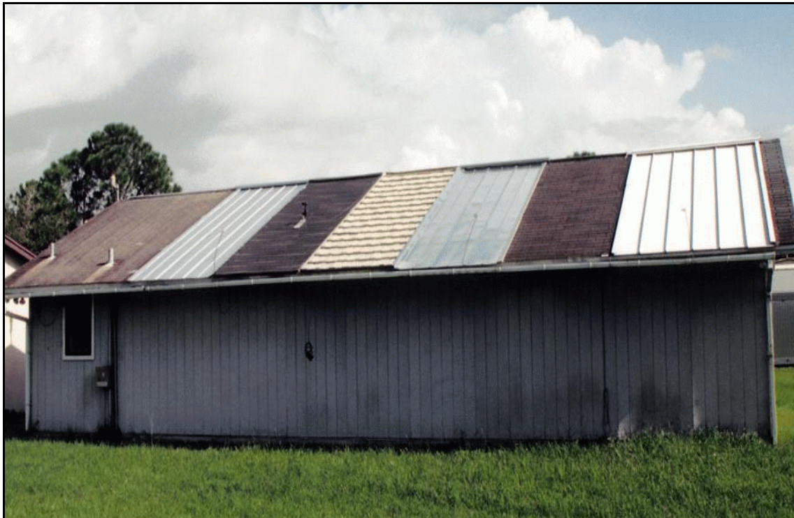
Figure 4. Flexible Roof Facility in summer 2002 configuration.
