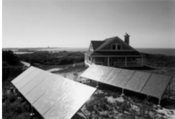
Figure 12.12 ASE America's Ground-Mounted Array
