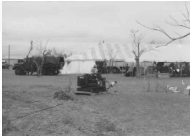
Figure 5.1 Military generator used in hurricane Andrew.
