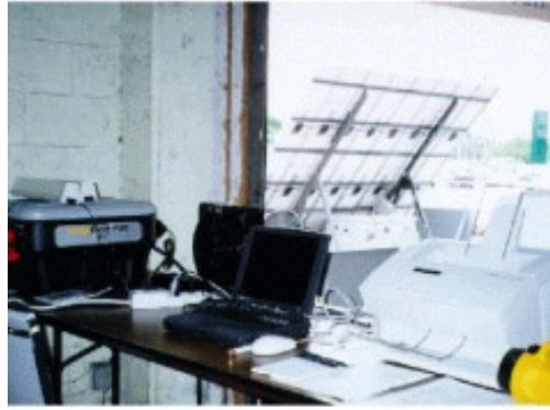
Figure 12.6 Some equipment being powered by the PV trailer at the Catholic Charities Distribution Center.
