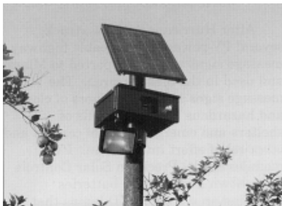
Figure 12.21 PV Security Lighting
