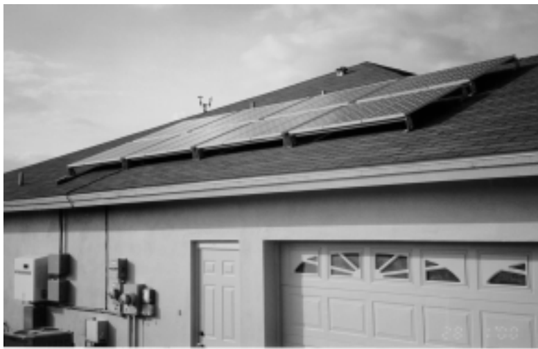
Figure13.1 Utility Interactive system.
