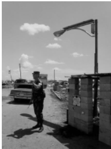
Figure 12.17 PV Lighting at Security Checkpoint
