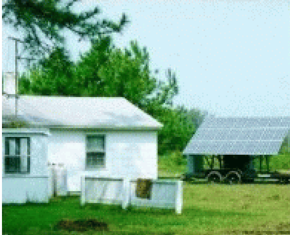
Figure 12.23 One of two FEMA PV trailer being used on Knotts Island after Hurricane Bonnie.
