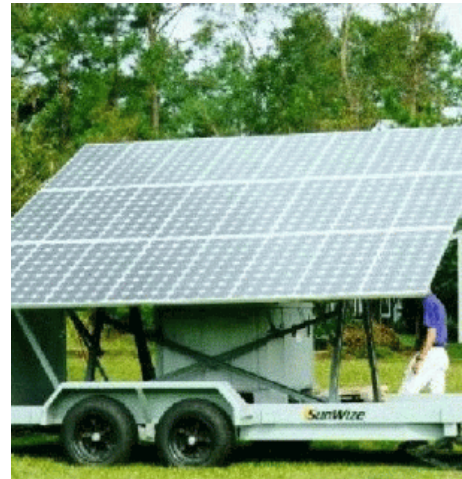
Figure 12.24 The second of two FEMA PV trailers being used on Knotts Island.
