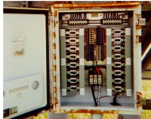
**Figure 25. System 6 Source Circuit Junction Box**
