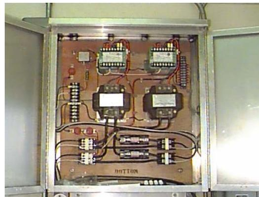
**Figure 8. System 1 AC Junction Box**
