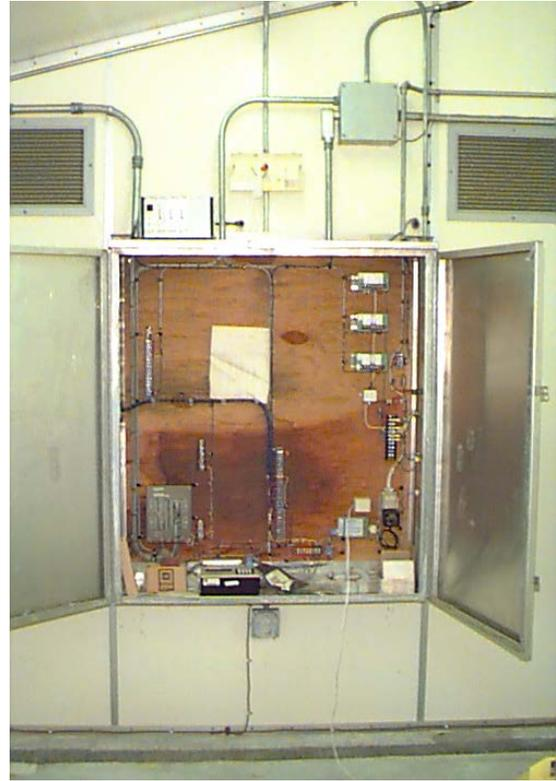
**Figure 32. Data Acquisition System**
