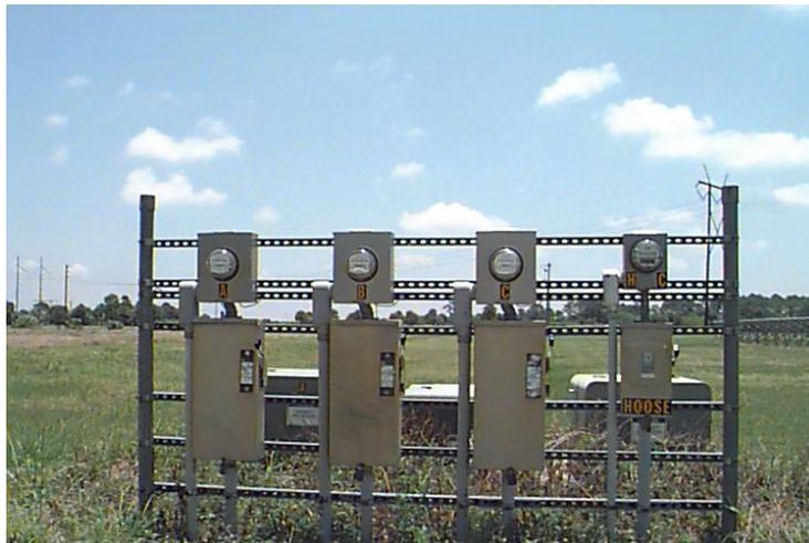
**Figure 4. Grid Interconnect and Metering Equipment**
