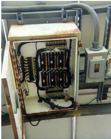
**Figure 18. System 4 Source Circuit Junction Box**
