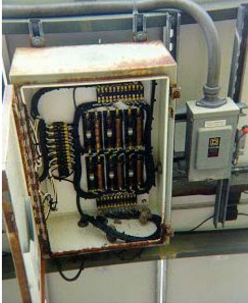
**Figure 14. System 3 Source Circuit Junction Box**
