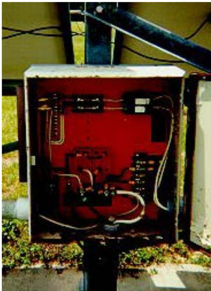
**Figure 10. System 2 Source Circuit Junction Box**
