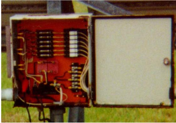
**Figure 6. System 1 Source Circuit Junction Box**
