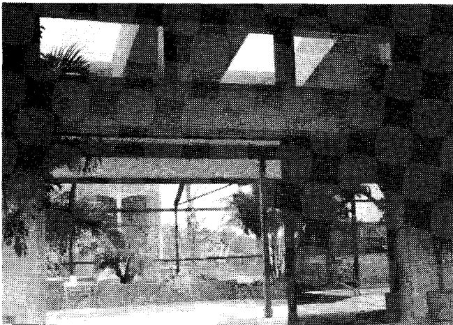
Skylights should be located on a porch rather than in the conditioned space.
