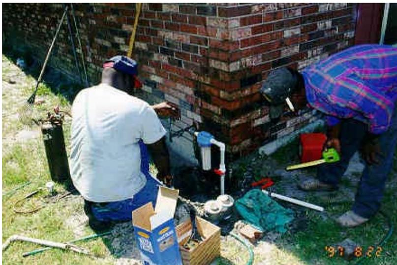
Figure 2.1-5. Whole house filter being installed.
