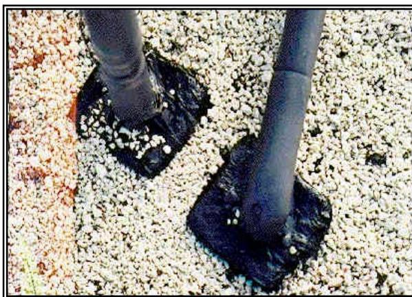
Figure 2.3-1. Pitch pan filled with bitumen.
