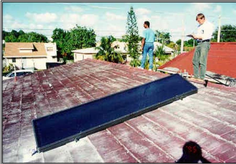
Figure 2.0-1. Twenty-square-foot collector installed on tile roof.
