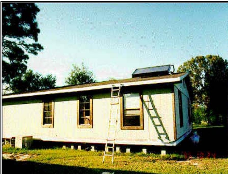
Figure 2.2-3. ICS system inadvertently installed on mobile home.
