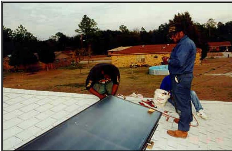
Figure 2.1-3. Local plumber installing ICS system.
