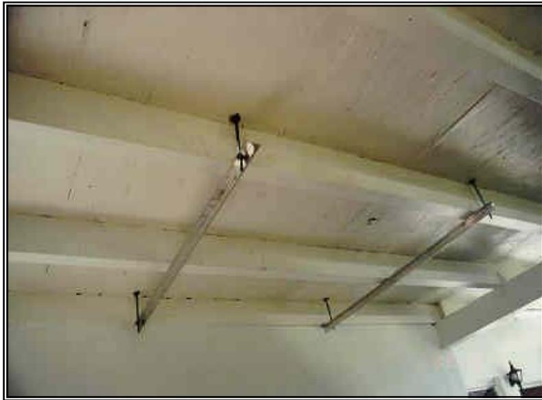
Figure 2.2-2. Spanner mounting of solar collector.
